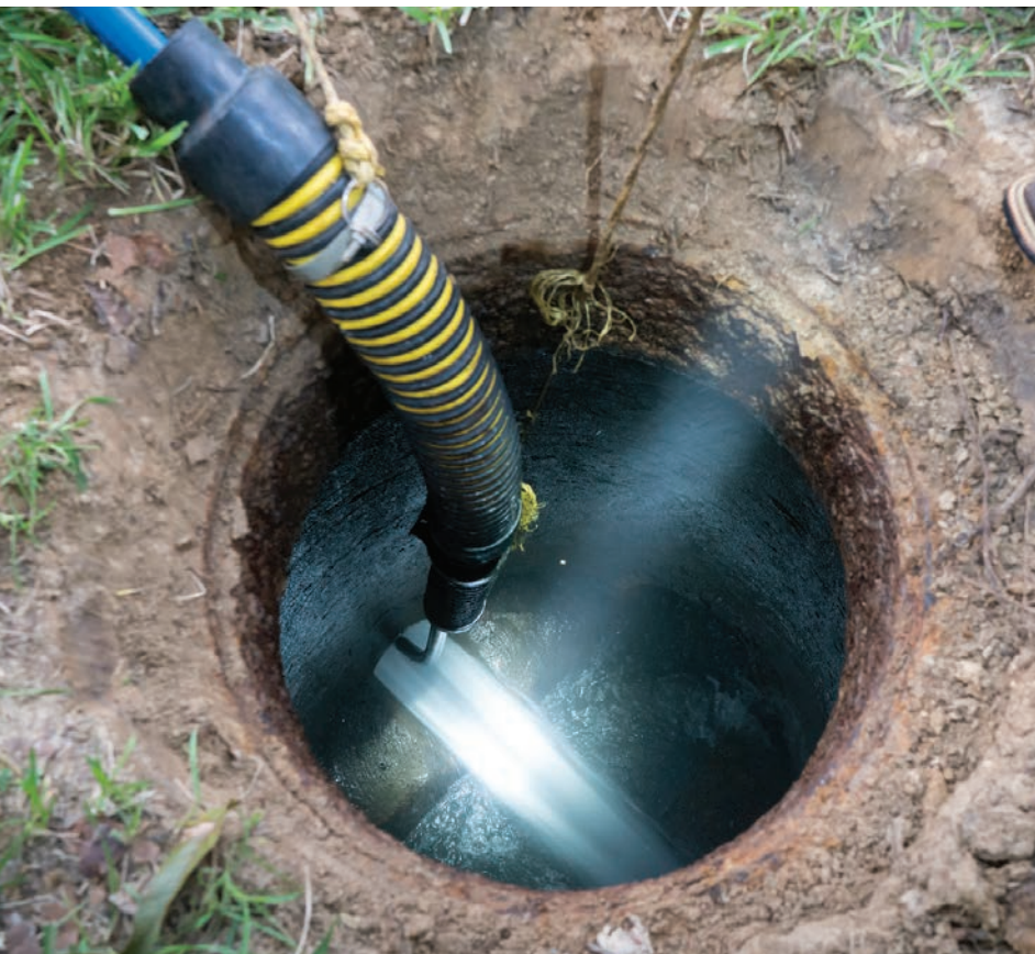
ABOVE Donald Browder (left) and Dalrone Kinchin of Compliance EnviroSystems use an easement machine running off a Vac-Con combination truck to jet a sewer line in Baton Rouge, Louisiana.
