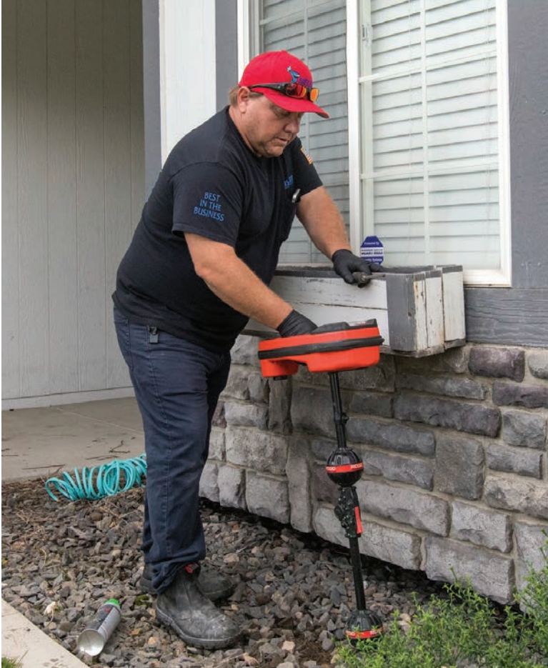
ABOVE & >>> Absolute Drain owner Mickey Castonguay uses a RIDGID NaviTrack locator to trace the path of a sewer lateral outside a customer's home.
