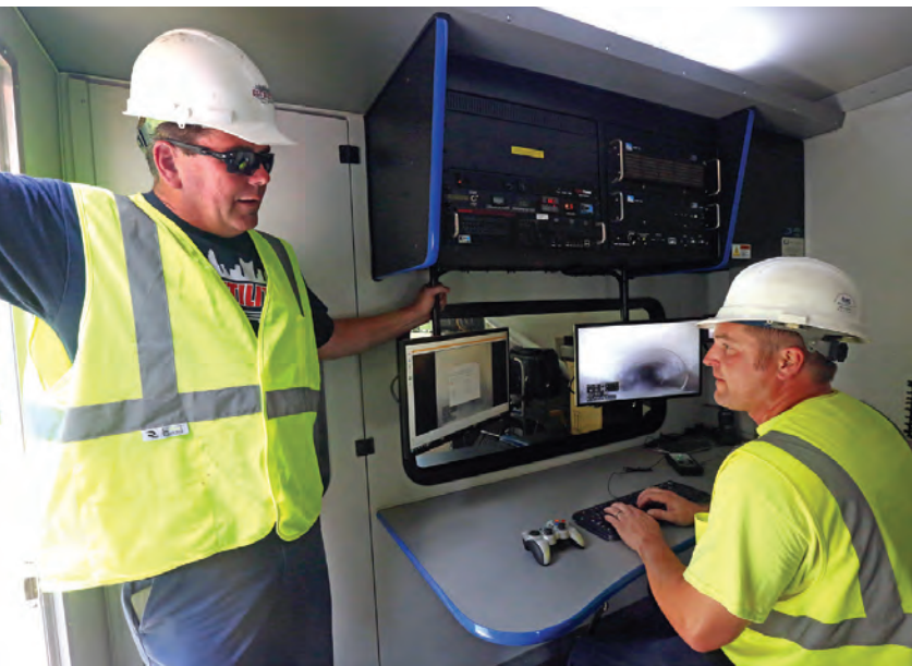
Owner Chuck Lang (left) speaks with camera technician Kevin Lyons about a lateral assessment job in the control room of the inspection van.
