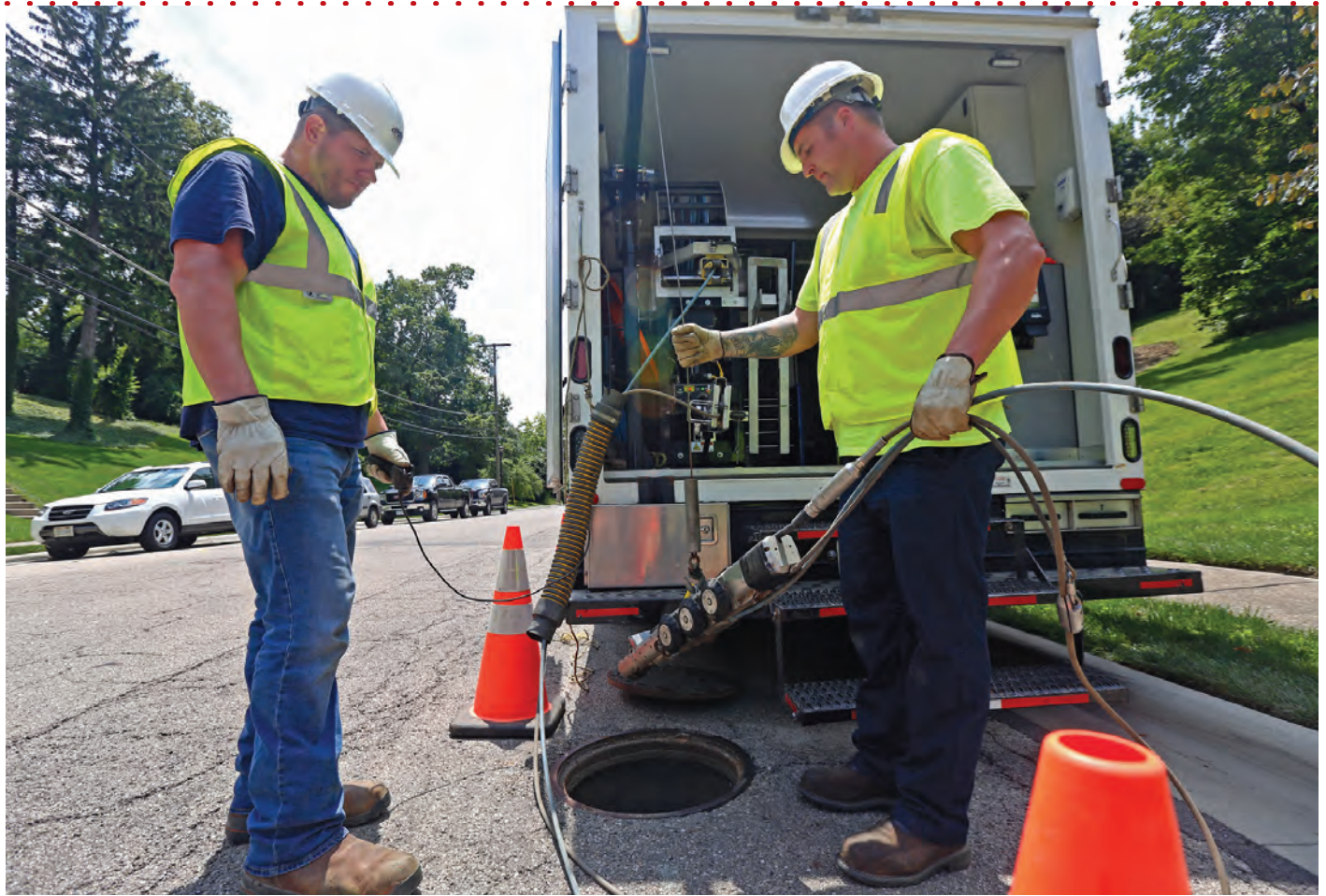
◀◀ Michael Snider of Chuck's Septic Tank Sewer & Drain Cleaning operates the controls on a Harben trailer jetter while clearing a drainline.
