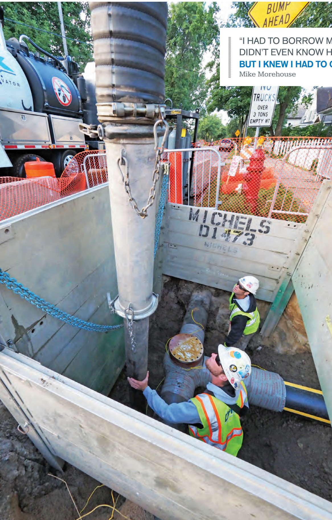
ABOVE Davids Hydro Vac operator Randy Becker guides the Vactor HXX hydroexcavator’s boom inside a shored trench while he and laborer Nate Otto clear the site for a utilities relocation project.
