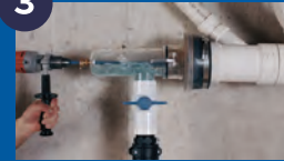
CUT HOLE IN DRAIN CAP
