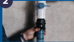
ATTACH DRAIN HOSE
