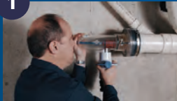
CLAMP TO CLEAN OUT DRAIN
