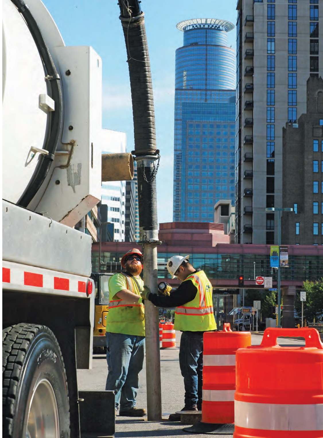
Davids Hydro Vac operator John Shuneman (left) and laborer Jason Bauer vacuum debris from a utility line cleanout in downtown Minneapolis.
