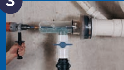
CUT HOLE IN DRAIN CAP
