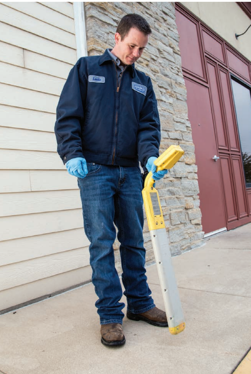
<< Louis French traces the path of a sewer lateral with a UEMSI locator.
