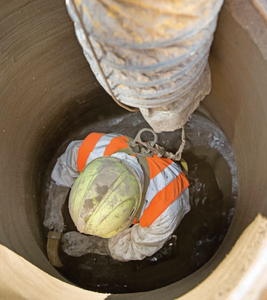
<< Felipe Servin brushes the final coat of Strong Seal MS- 2C cement liner inside a manhole.
