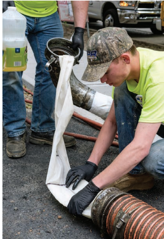
Eric Poteet feeds a liner into the inversion tube for installation.
