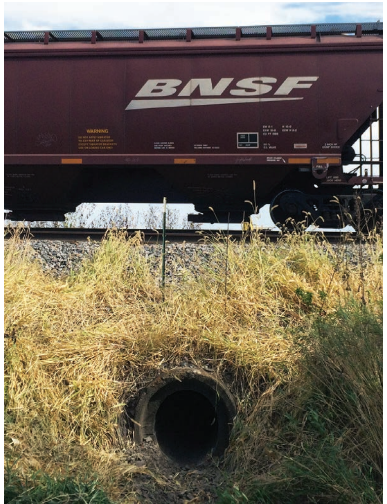
The point repairs have both an H2O live load rating for use under highways and a Cooper 80 live load rating for use in rail beds, independent of the existing pipe.
