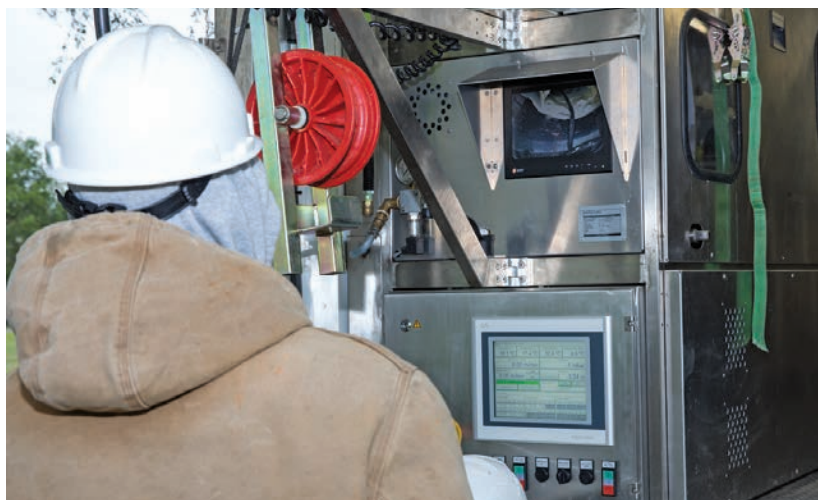
BELOW Malcolm Brumley monitors the ProKASRO light train during the curing process.
