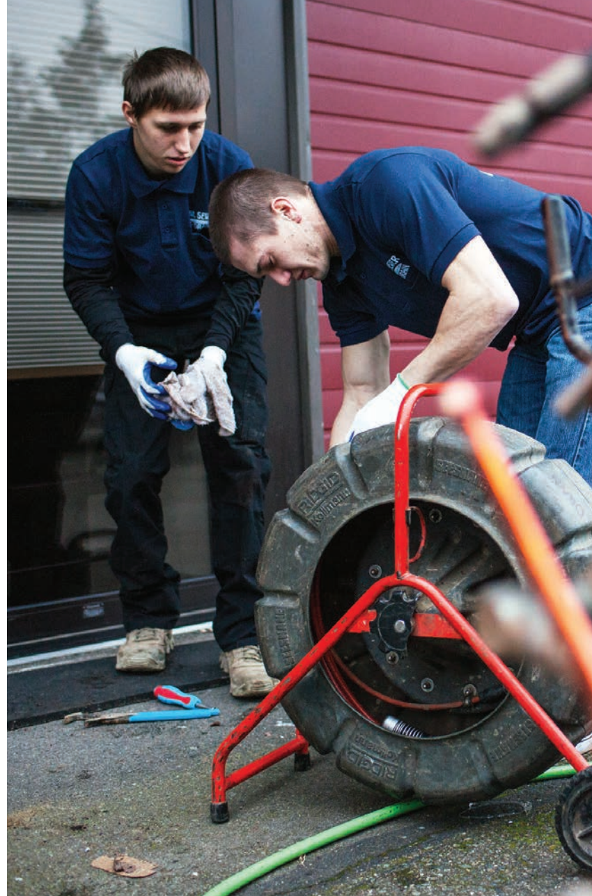
ABOVE Derek Thomas pulls hose off the reel and keeps a hand on the trailer jetter controls while clearing a commercial sewer line blockage.
