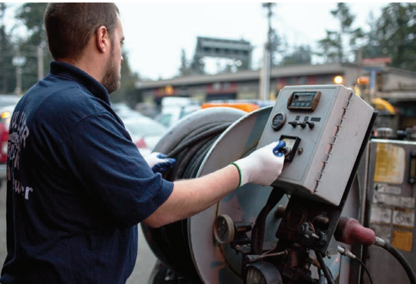
ABOVE Derek Thomas pulls hose off the reel and keeps a hand on the trailer jetter controls while clearing a commercial sewer line blockage.
