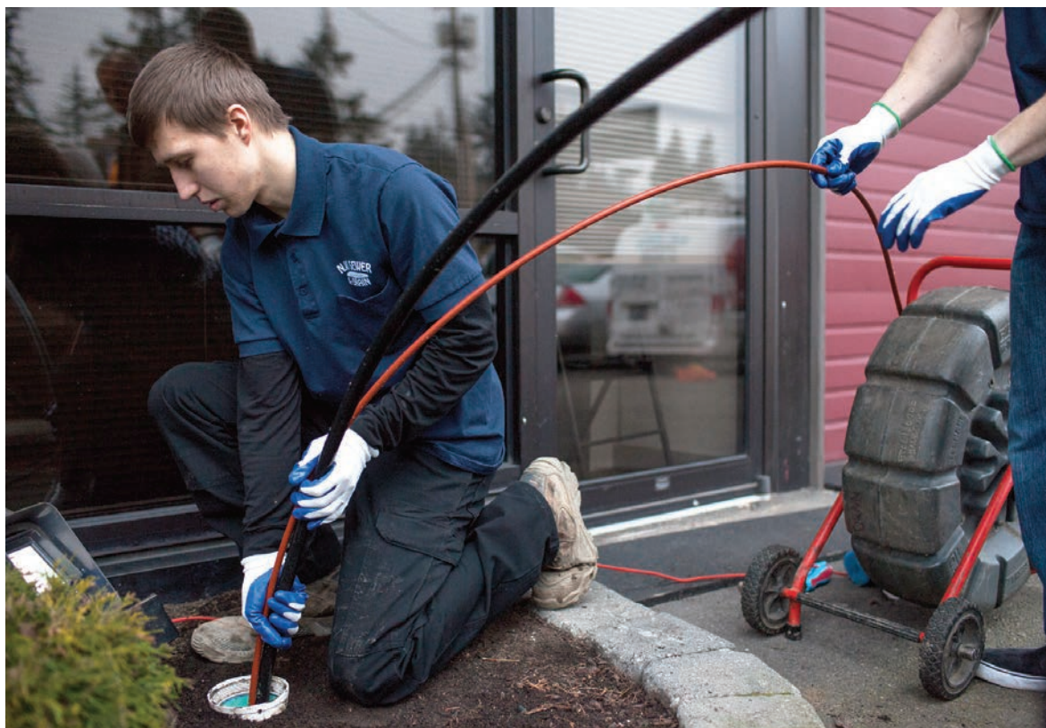
◀◀◀ Josh Schemmel keeps an eye on the monitor as he feeds the SeeSnake cable into a clean-out behind the jetter hose.
