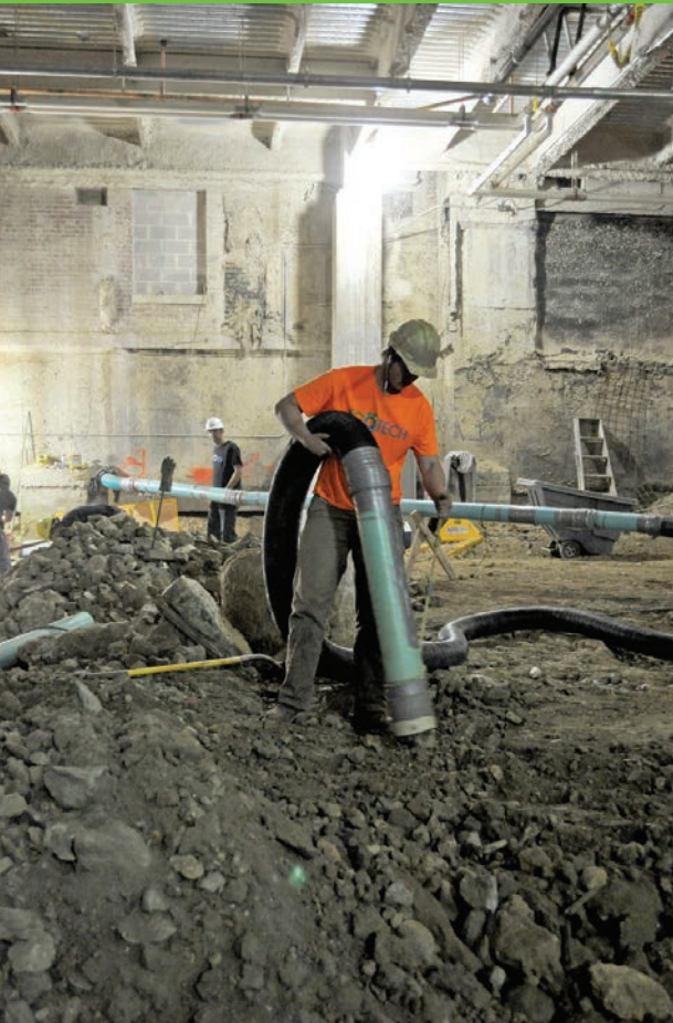
<< A crew member from Ecotech Hydro Excavation carries a heavy-duty vacuum hose — with a short section of PVC pipe attached for added durability — through the basement of the hospital in Philadelphia.
