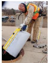
debris/blockage within the pipeline. Forward-looking sonar continuously updates, has a field of view of 120 degrees and can see objects up to 50 feet ahead of the vehicle. The company was able to obtain real-time feedback of the vehicle's progress to ensure it did not swim past the valve. The forward-looking sonar also filled in the gaps between profiles to ensure they were not missing any areas of higher debris between scans and abnormalities.
