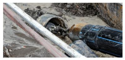
New HDPE pipe, attached to the bursting head, is pulled into the host pipe.
