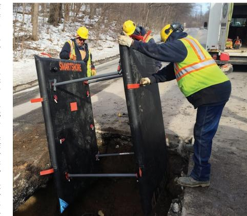
With each section weighing only 29 pounds, Smartshore is easy for workers to set in place and transport.
