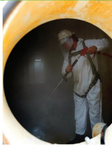
ABOVE: A technician cleans the inside of a steel tank with a high-pressure waterblasting
