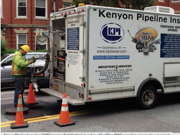
Kenyon Pipeline Inspection CCTV operator Todd Kuklinski launches a RapidView IBAK inspection camera into a municipal
