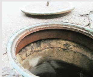
Concrete ADJ Rings Installed 1997
