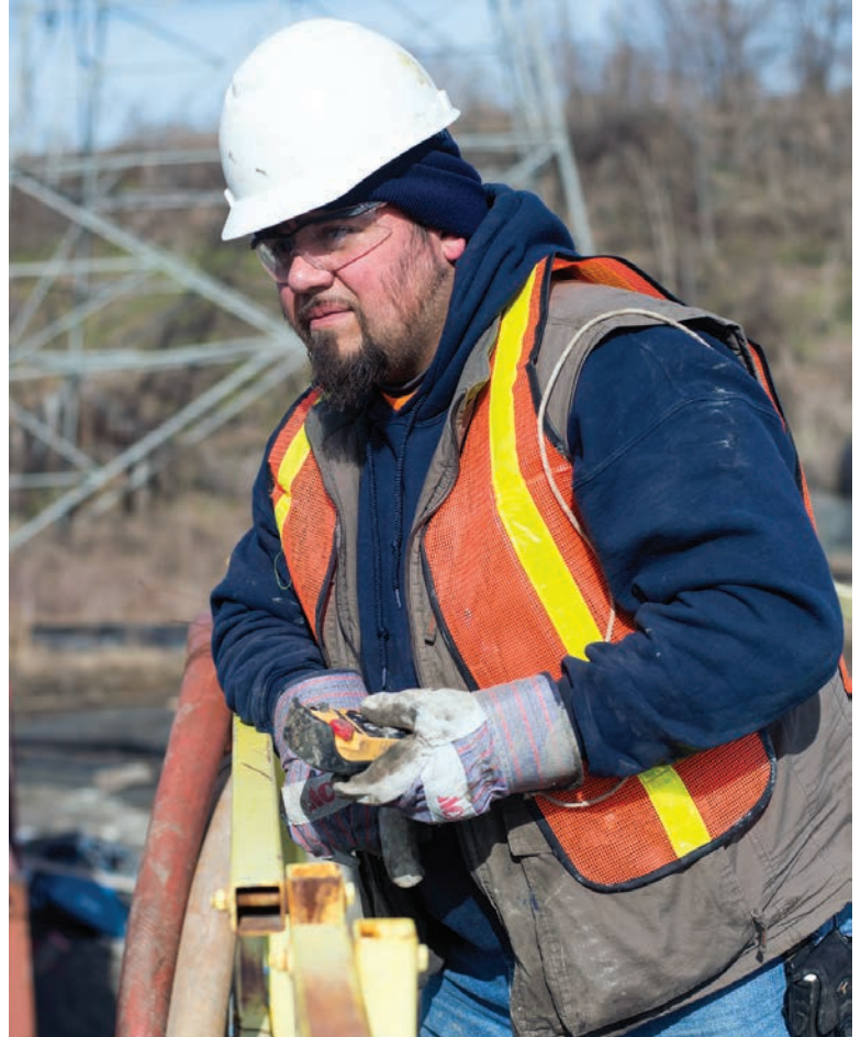
Backlund Plumbing technician Johnny Compos uses a remote control to guide a hydroexcavation boom at the Leavenworth Lift Station.
