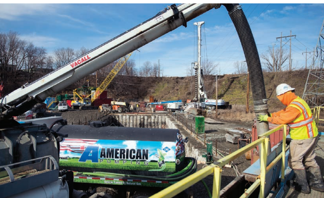
Backlund Plumbing technician Jamey Severn guides the boom from a Vacall AllExcavate hydroexcavator into a Rain for Rent dewatering tank at the Leavenworth Lift Station replacement project in Omaha, Nebraska.
