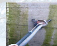
Air Recovery Works on Walls
