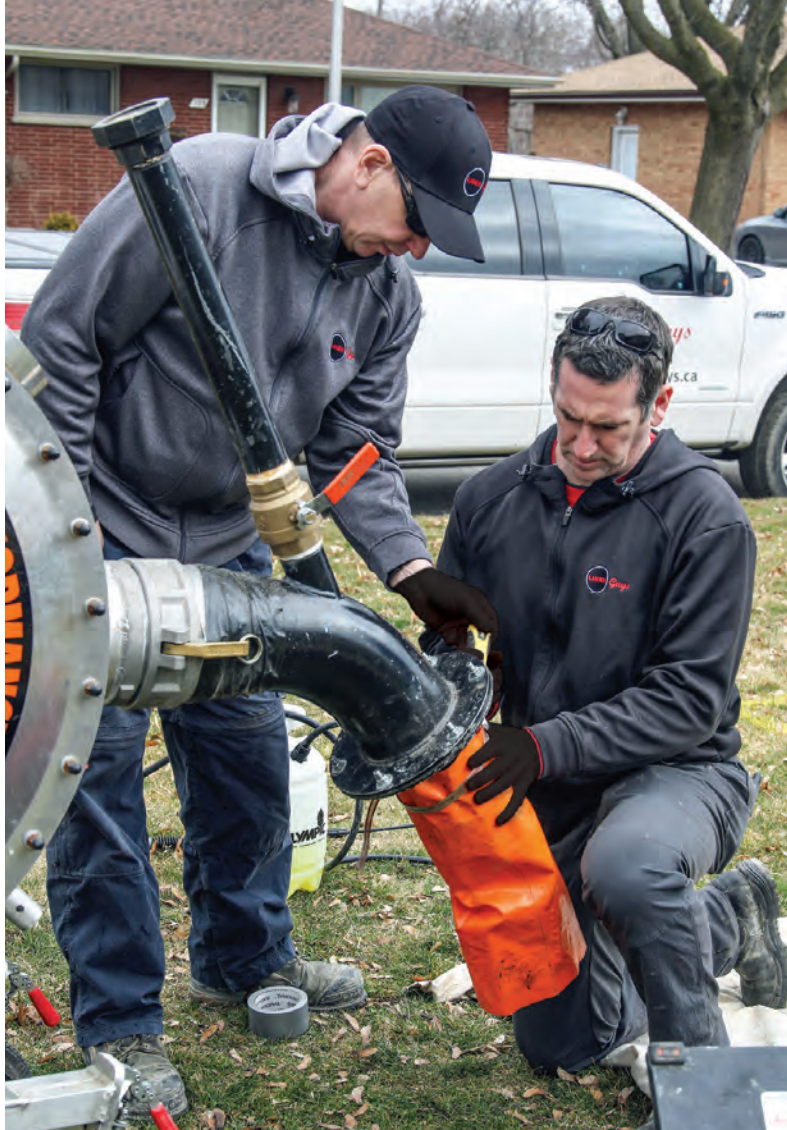
Dennis Matthew (left) helps Mike Rodger get set up to shoot a liner into a 4-inch sewer lateral.
