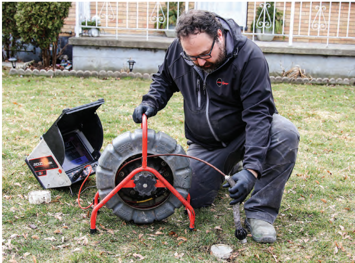
Steve Stefanidis does a post-lining inspection with a RIDGID SeeSnake camera and CS10 color monitor.
