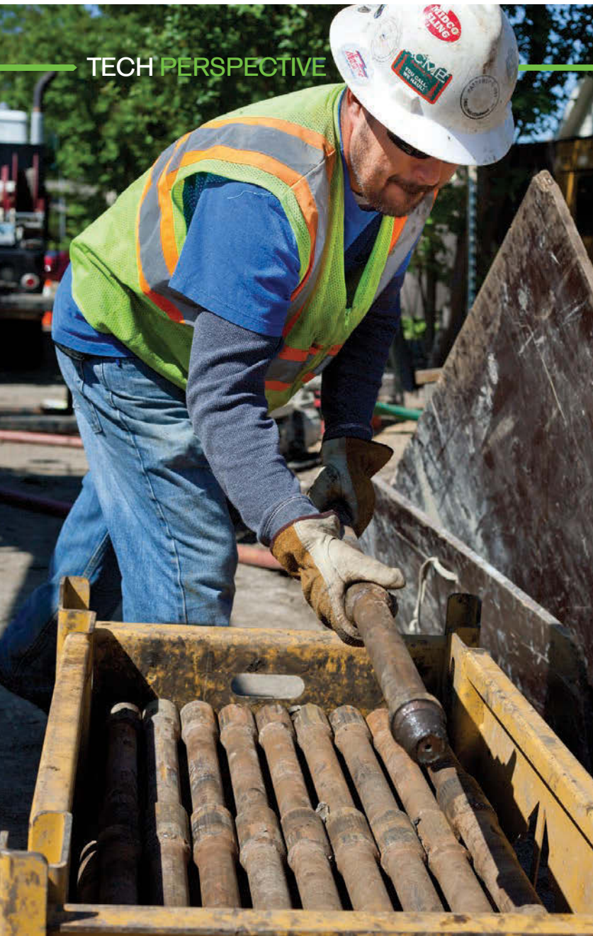
<< LEFT: A worker stows rods from a pneumatic pipe bursting system as the new pipe is pulled into place. Pneumatic bursting systems use an air compressor to operate the bursting tool, so maintaining the air hose is critical.
