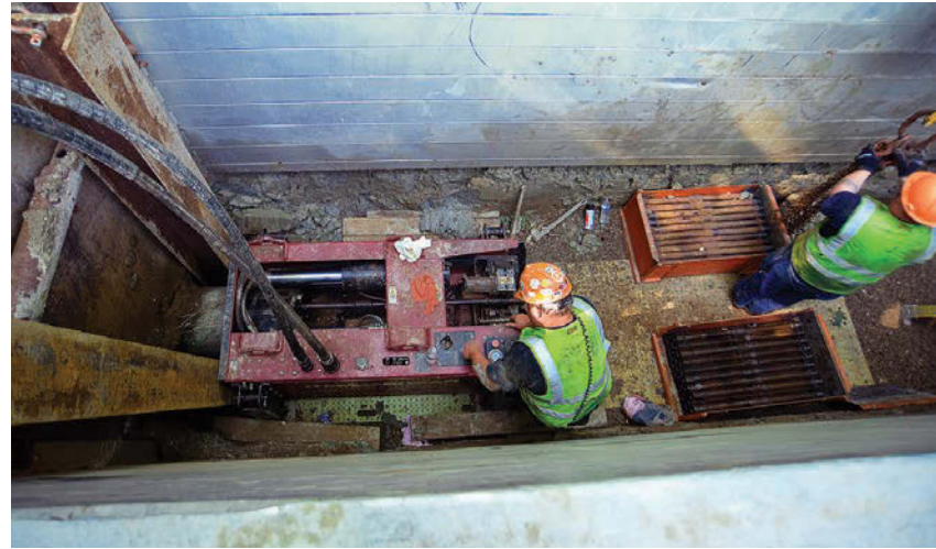
<< LEFT: A worker stows rods from a pneumatic pipe bursting system as the new pipe is pulled into place. Pneumatic bursting systems use an air compressor to operate the bursting tool, so maintaining the air hose is critical.
