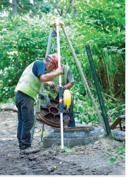
Mike Cram and Dave Bilodea set up for a confined-space entry at a manhole along the path of a pipe bursting project.
