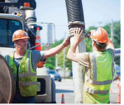
Andy Bryant (right) attaches an extension tube to the vacuum boom on a Vactor 2116 as the crew prepares to clean a 48-inch stormwater outfall pipe.
