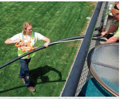
Allied Plumbing & Pumps co-owner Ron Smiley (left) works with Korey Kase to measure and cut a new length of pipe for a pipe bursting job.
