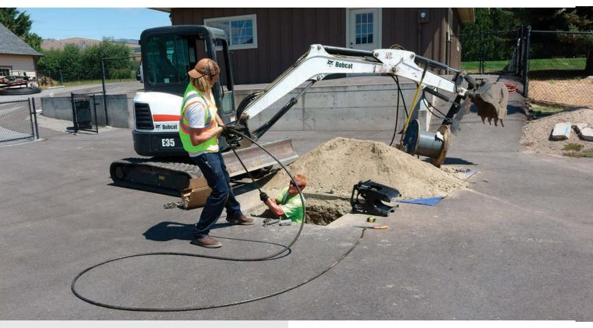
ABOVE: Ron Smiley (left) and Korey Kase pull the slack out of the cable before hooking up the hydraulic pipe bursting head to pull in a new wastewater line.
