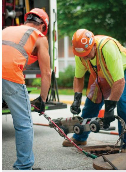
Larry Houle (right) and Billy Timberlake lower an Aries Badger transporter and camera into a manhole to inspect a brick sewer main.
