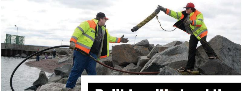
**ABOVE:** Dylan Sigfrids (right) of Great Lakes Pipe Service tosses a Tiger Tail to his dad as they set up to jet a stormwater line along the shore of Lake Superior in Duluth, Minnesota.
