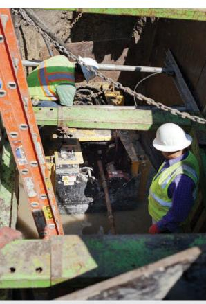
No-DigTec workers operate a HammerHead hydraulic pipe bursting unit in the receiving pit, pulling in 5,000 feet of new 8-inch PVC pipe.
