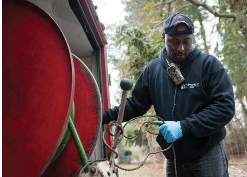
ABOVE: Wisler Sanon uses rope and a plastic tube to guide a 1/2-inch jetting hose where it needs to go inside a sewer lateral at a home in Ewing, New Jersey. Because the blockage was extensive, Sanon decided to treat the blockage from both inside and outside of the home.
