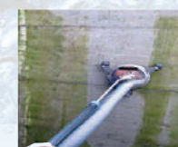
Air Recovery Works on Walls
