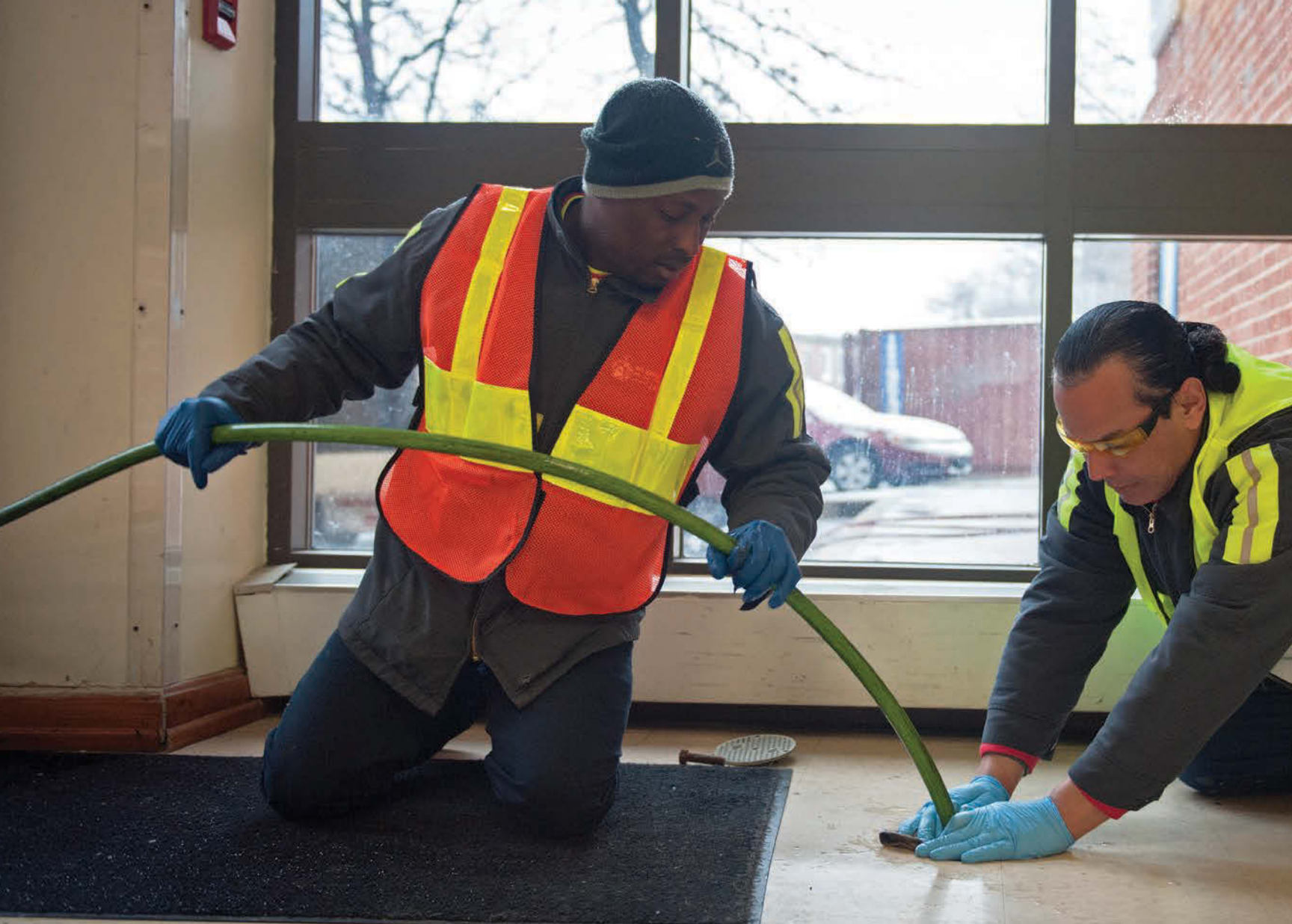
ABOVE: All Service Plus owner Wisler Sanon (left) and drain specialist Mario Condis use a 1/2-inch hose off the truck-mounted jetter (US Jetting) to clean a drain inside an apartment complex in West Philadelphia. Condis holds a cloth over the drain opening to prevent debris from splashing into the hallway when it clears.
