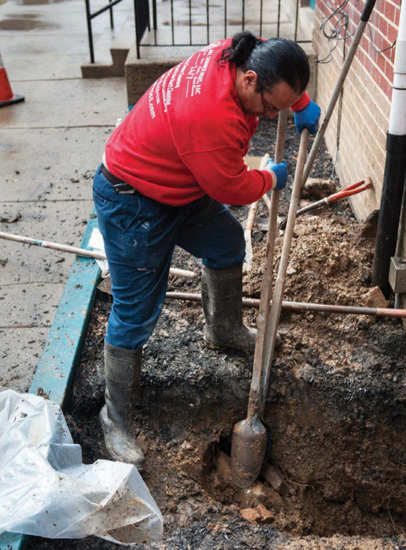
ABOVE: Wisler Sanon uses rope and a plastic tube to guide a 1/2-inch jetting hose where it needs to go inside a sewer lateral at a home in Ewing, New Jersey. Because the blockage was extensive, Sanon decided to treat the blockage from both inside and outside of the home.
