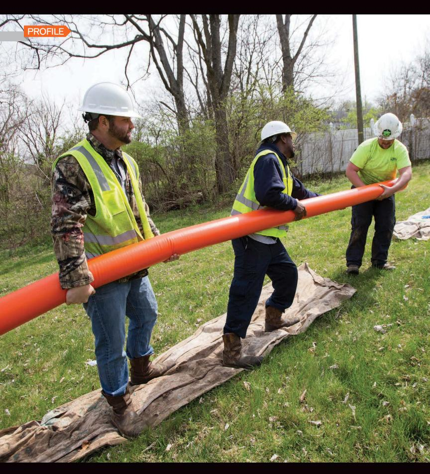
Jake Johns, Tyrone Walls and Brent Faust (from left) of BLD Services prepare a liner for a lateral rehabilitation project.
