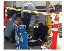
pressurized pipe inspection and leak detection system designed for harsh environments.
