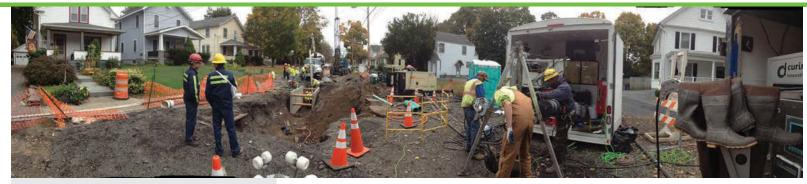
Members of the Kingston Department of Public Works (left) excavate to repair an 8-inch sewer that collapsed adjacent to the main sinkhole. The entry supervisor and attendant (right) from Precision Industrial Maintenance in Schenectady, New York, monitor a confined space entry.
