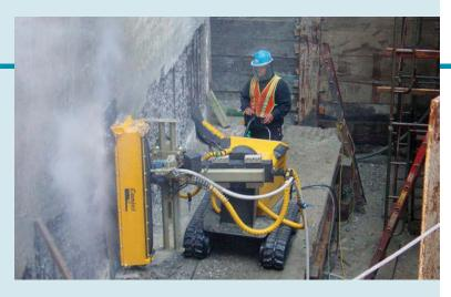
Attachments include the standard surfacing tool for flat structures, horizontal and vertical; the surface preparation tool for removing the topmost layer of concrete and steel; and the ship cleaning tool for removing paint, rust and barnacles from hulls and other curved surfaces.
