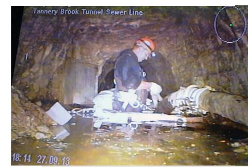
ABOVE: Tim Nappi stands in the Tannery Brook Tunnel as the crew prepares to line the 24-inch sanitary sewer.
