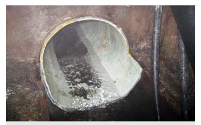
ABOVE: After curing the 24-inch SAERTEX fiberglass-reinforced plastic liner, the ends were cut flush with the headwall and floor of the tunnel.
