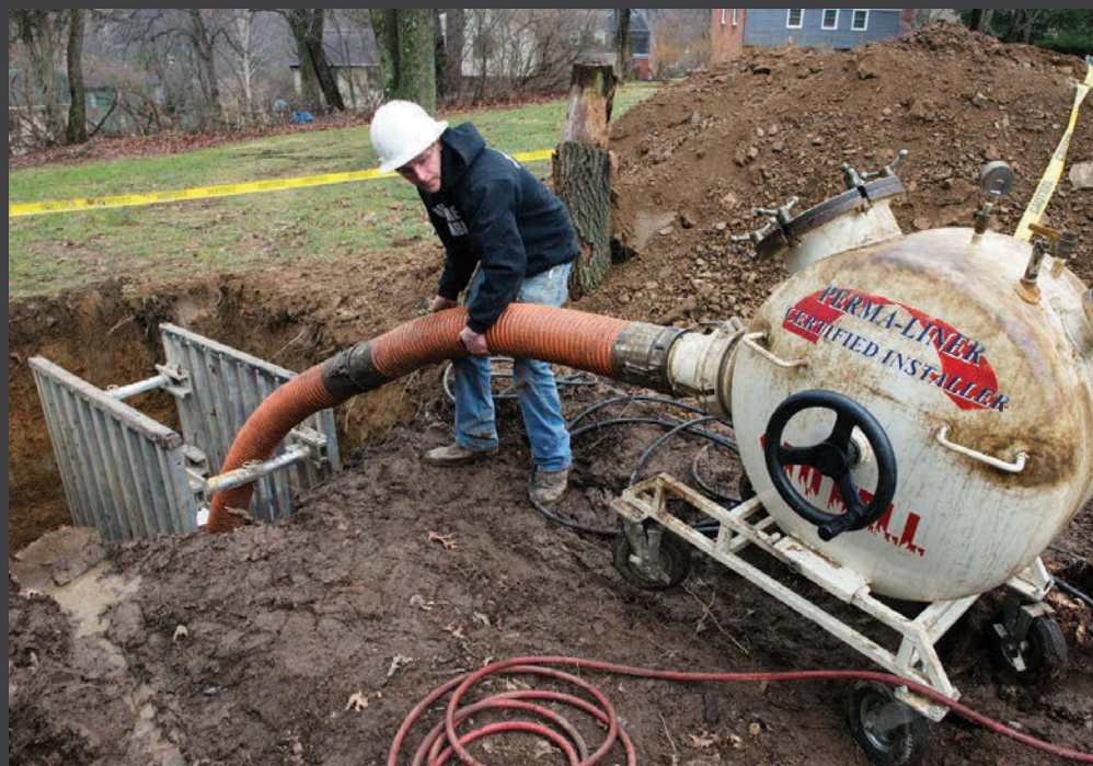
Dylan Belfiore guides the Perma-Lateral inversion unit at the entry pit on a lateral relining job.
