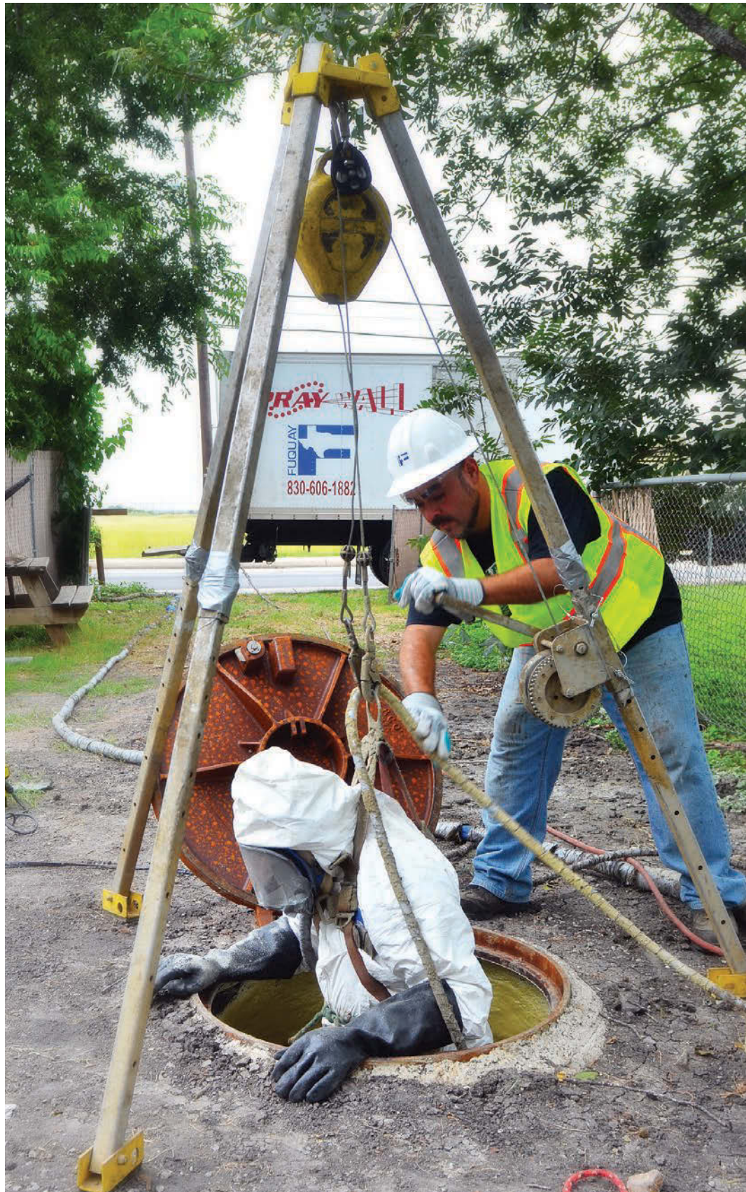
ABOVE: Manhole rehabilitation technician Sergio Alvarez mixes grout for a manhole rehabilitation job in San Antonio.
