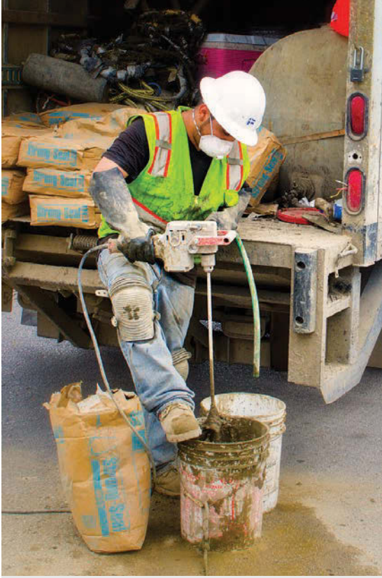
ABOVE: Manhole rehabilitation technician Sergio Alvarez mixes grout for a manhole rehabilitation job in San Antonio.
