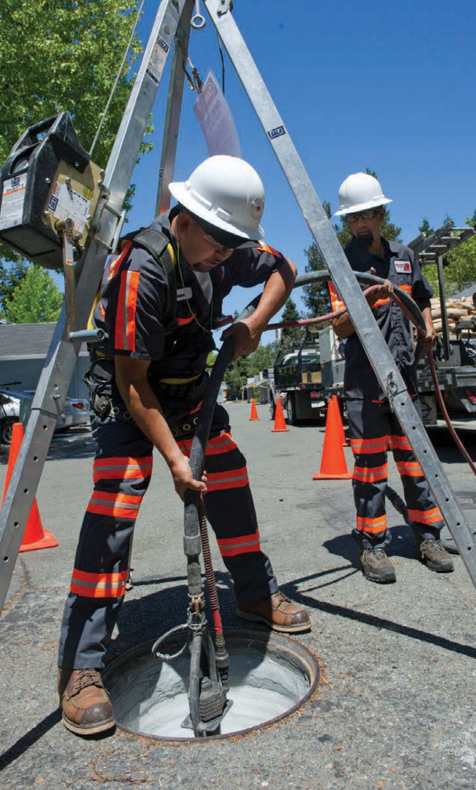
LEFT: Jesus Uriarte lowers a modified Madewell Spin Caster into a manhole during a rehabilitation project. BELOW TOP: The Spin Caster sprays an even coat of composite liner around the interior of the manhole. BELOW BOTTOM: The rehabilitated manhole lined with Mainstay composite material.
