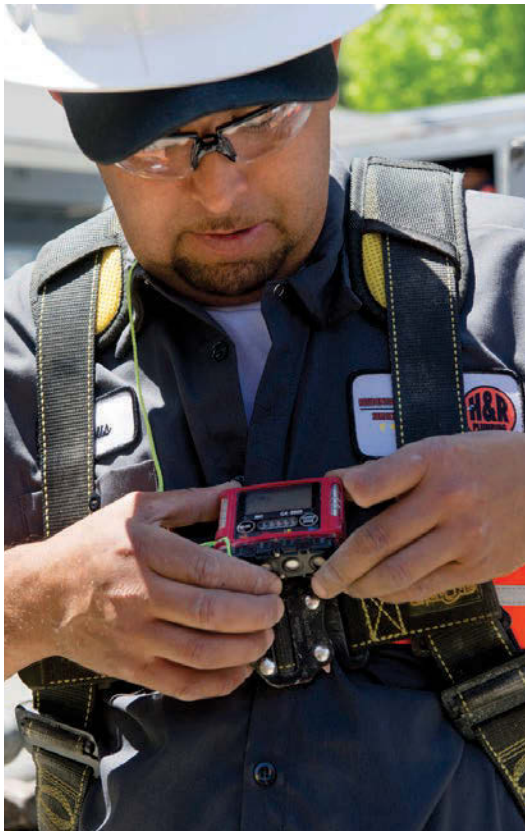
Jesus Uriarte checks the gas monitor affixed to his confined-space entry gear while on a manhole rehabilitation job.
