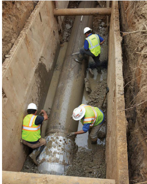
LEFT: Unable to dump to the side, the excavator operator swings another bucketful behind the machine in the constricted work area of Stone Creek Park in Fort Worth, Texas. (Photo courtesy of John Newell) BELOW: No-DigTec workers separate the bursting assembly from the HDPE pipe in the 60-foot-long, 15-foot-deep pit. (Courtesy of John Boykin)
