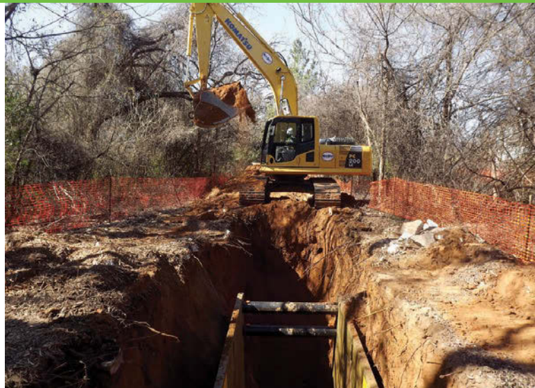
LEFT: Unable to dump to the side, the excavator operator swings another bucketful behind the machine in the constricted work area of Stone Creek Park in Fort Worth, Texas. (Photo courtesy of John Newell) BELOW: No-DigTec workers separate the bursting assembly from the HDPE pipe in the 60-foot-long, 15-foot-deep pit. (Courtesy of John Boykin)
