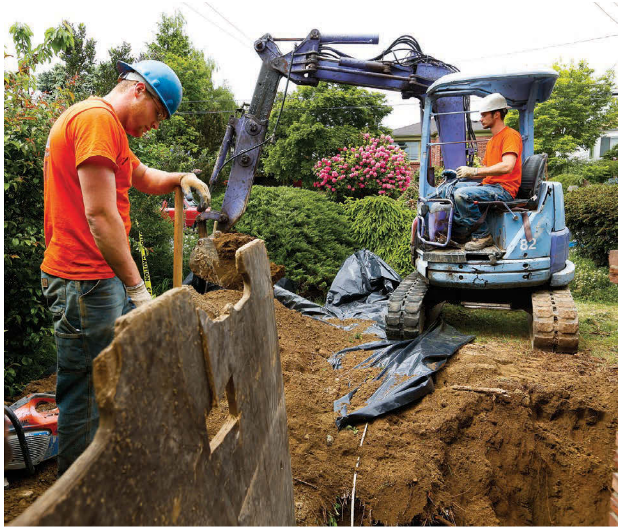
ABOVE: Technicians Luke Boer (left) and William Coffman excavate a residential lateral line for repair. BELOW: Technicians Joshua Stubbs (left) and Austin Berg take measurements while working on a lateral line replacement job.
