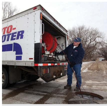
Pat Brown uses a truck-mounted jetter (US Jetting) to clear sludge and debris in a sewer line.
