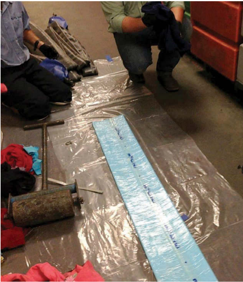
A roller (left) forces epoxy into the liner.
