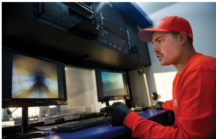
Express Sewer & Drain camera operator Alan Smith prepares the CUES camera and monitors an inspection job inside the CCTV truck.
