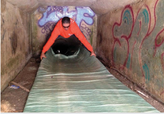
ABOVE: Miguel Romero of Express Sewer & Drain guides liner into a 30-inch storm drain culvert on a recent CIPP lining project. >> Dillon Moore and William Blake unload liner from a refrigerated truck and feed it into the culvert. (Photos by Bill Heinselmann)
