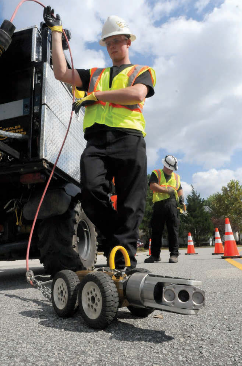
LEFT: Cody Thompson readies the camera rig to inspect a stormwater pipe. BELOW: Working from the Kubota RTV 900, technicians Cody Thompson, Dylan Williams and Trevor McGhee (from left) pull the inspection camera back through the manhole.
