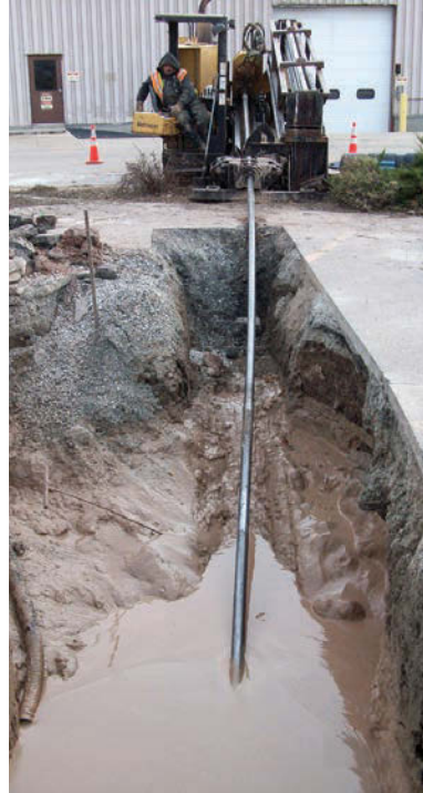
ABOVE: Eric Feucht (left) uses a walkie-talkie to direct the excavator operator as he lowers the 26-inch fluted reamer into the pit. RIGHT: The Vermeer D50X100 rig with the trailing rod.
