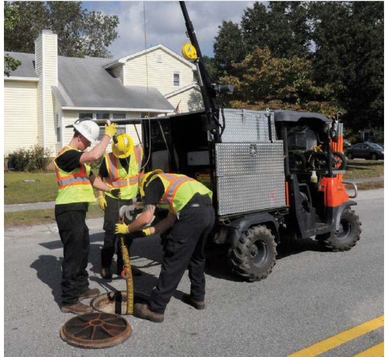
LEFT: Cody Thompson readies the camera rig to inspect a stormwater pipe. BELOW: Working from the Kubota RTV 900, technicians Cody Thompson, Dylan Williams and Trevor McGhee (from left) pull the inspection camera back through the manhole.
