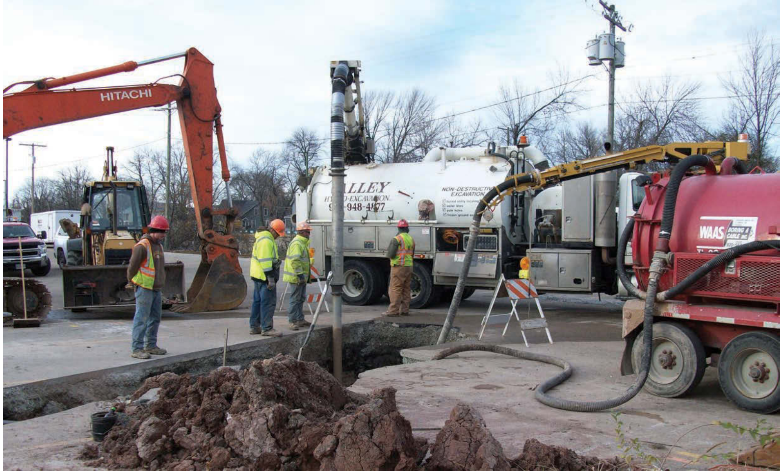
ABOVE: A hydroexcavator from Valley Hydro-Excavation in Campbellspport, Wis., helps a Waas vacuum tank trailer pump drill fluid from the exit pit. RIGHT: The custom-built 20-inch rock reamer has six carbide Tri-Cone bits with large cone offsets, chisel-shaped inserts, and irregular tooth spacings. Fins ahead of the reamer keep it centered in the smaller hole.
