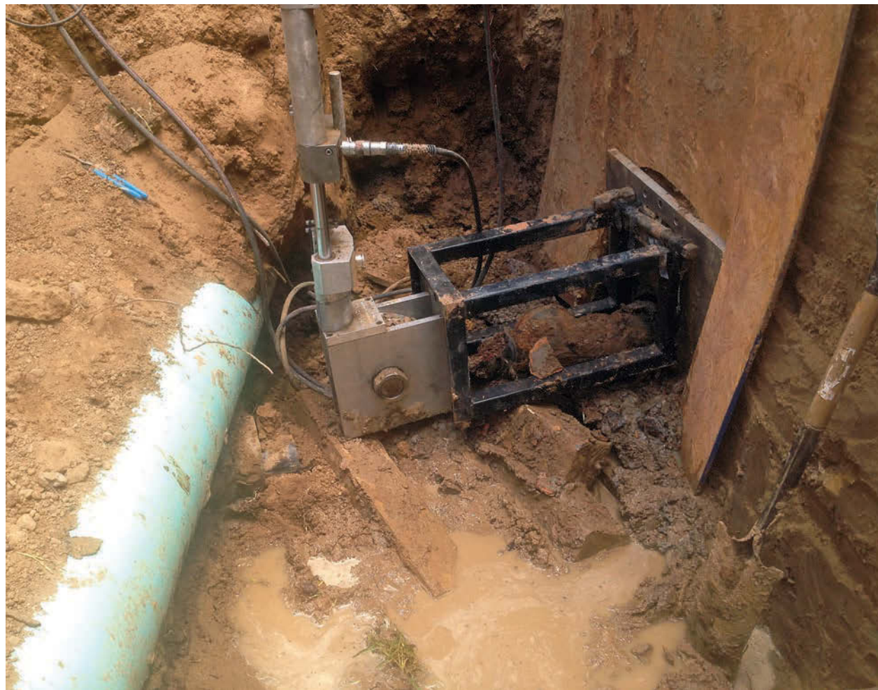
ABOVE: The TRIC C20 pipe bursting system, rated for 8,000 psi, sits at the bottom of the 8-foot-deep pulling pit next to the water main. Operations Manager Michael Smith used a Sharp Shooter drain spade to cut crisp, straight walls against which to position the resistance plate. RIGHT: The 4-inch HDPE pipe advances through the enlarged holes in the concrete stormwater vault. Behind the pipe are two 36-inch diameter concrete drains. The original clay tile lateral switched to cast iron at this point.
