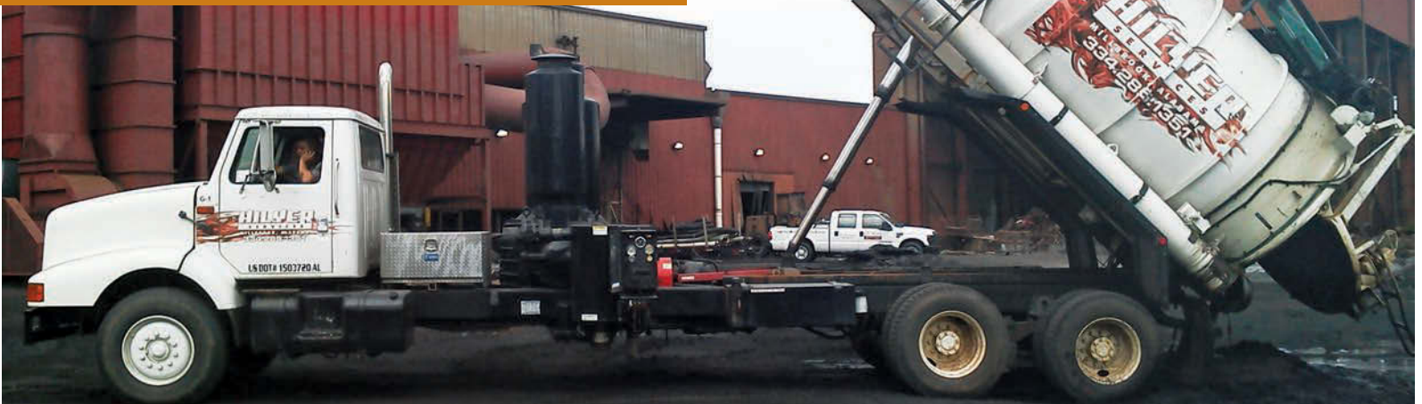
One of ATC/Hilyer Services’ Guzzler vacuum trucks offloads at a steel foundry in Marion, Alabama, where it was vacuuming liquid and dry material out of tunnels and pits and under conveyor belts.
