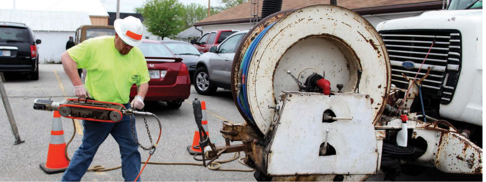
ABOVE: Scott Engineering employee Jerry Moore prepares to lower a camera into a sewer system during a job in Westport, Ind. LEFT: Jason Austin, right, feeds a camera into a sewer line as Dennis Denney, left, and Jerry Moore view the picture on a computer screen as they work on a lateral lining project.
