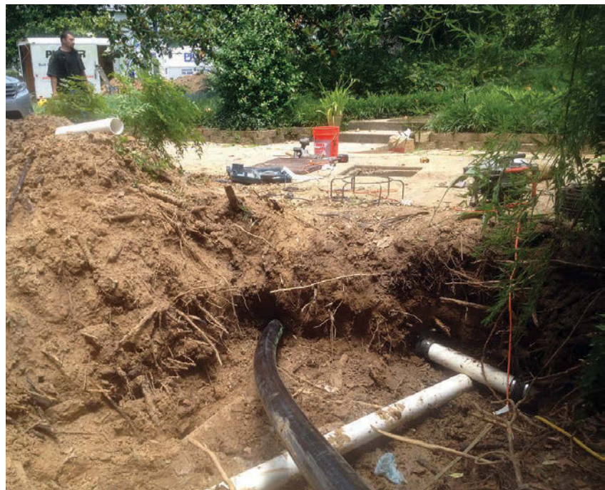
The 6- by 6- by 5-foot-deep entry pit was 6 feet upstream from the square stormwater vault with two 36-inch concrete drains.
