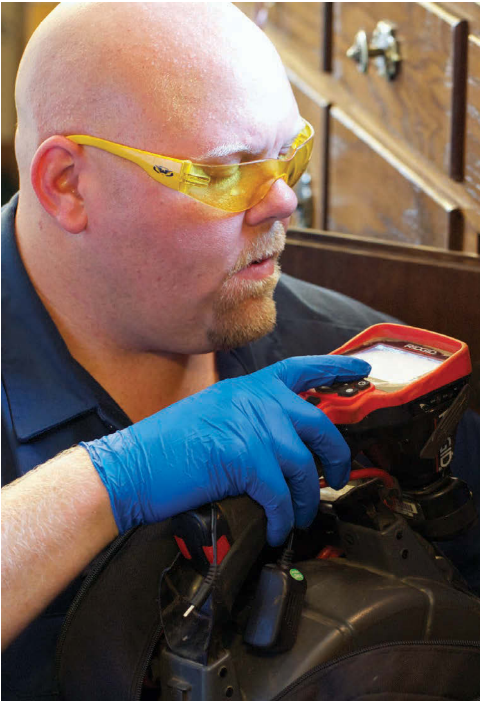
LEFT: Wesley Sanford uses a RIDGID SeeSnake to diagnose a drainline problem on a residential service call. All Ways relies on the RIDGID mini cameras for inspecting smaller lines.
