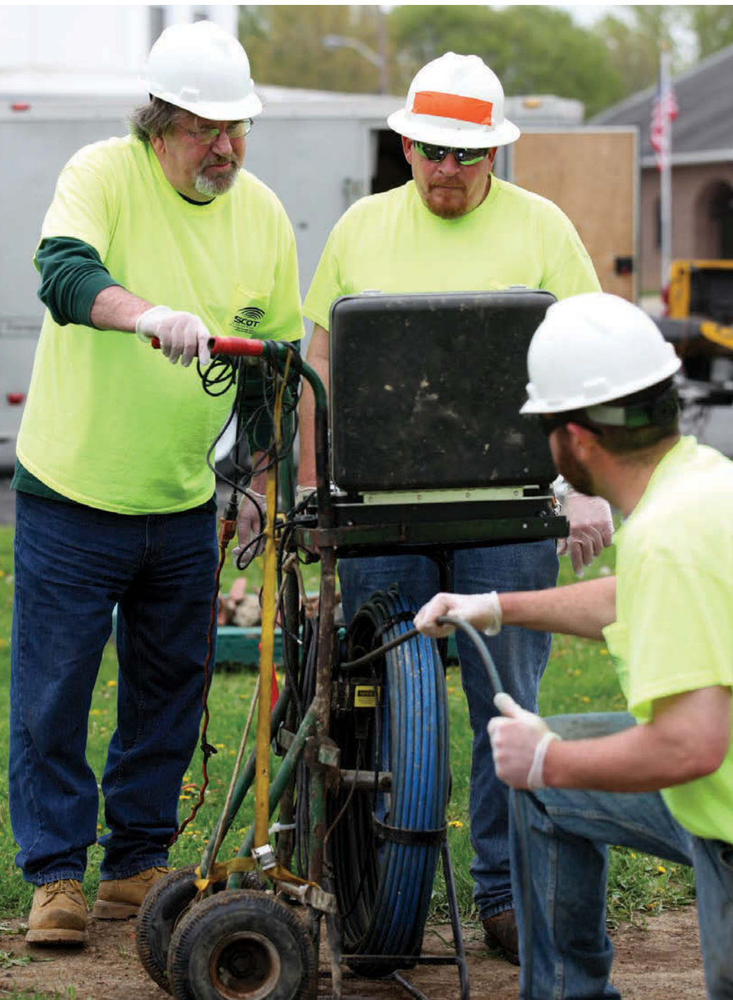
ABOVE: Scott Engineering employee Jerry Moore prepares to lower a camera into a sewer system during a job in Westport, Ind. LEFT: Jason Austin, right, feeds a camera into a sewer line as Dennis Denney, left, and Jerry Moore view the picture on a computer screen as they work on a lateral lining project.
