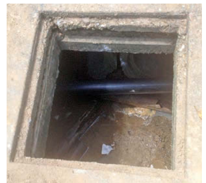
ABOVE: The TRIC C20 pipe bursting system, rated for 8,000 psi, sits at the bottom of the 8-foot-deep pulling pit next to the water main. Operations Manager Michael Smith used a Sharp Shooter drain spade to cut crisp, straight walls against which to position the resistance plate. RIGHT: The 4-inch HDPE pipe advances through the enlarged holes in the concrete stormwater vault. Behind the pipe are two 36-inch diameter concrete drains. The original clay tile lateral switched to cast iron at this point.
