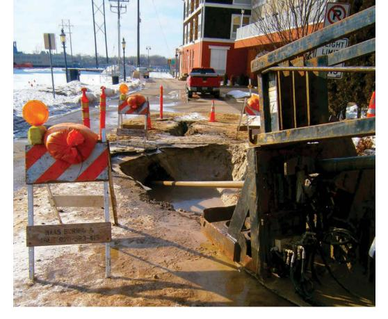
ABOVE: Waas staged the directional drill in front of the no parking sign by the hotel and restaurant. (Courtesy of Randy Waas) BELOW: Tim Stieve of Waas Boring and Cable feeds the 1.25-inch HDPE tubing into the exit pit at the back of the locktender house, as two other laborers in the background unroll it from the spool and work out the kinks. (Courtesy of Jim Kneiszel)
