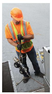
Jake Kenyon removes a crawler camera from a catch basin after performing a CCTV pipe inspection. (Photography by Jason McKibben)
