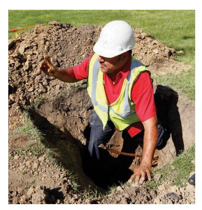
Martin Salazar pulls a new 60-foot piece of 3/4-inch copper roll pipe through the exit pit on a job in Washington Township, Ohio.
