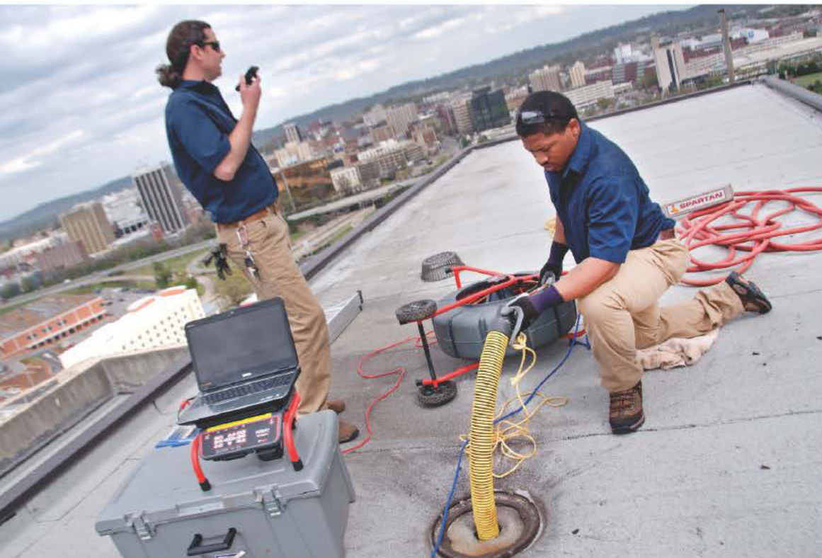
Danzel Owens sets up a SeeSnake reel for the rooftop inspection.
