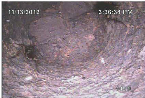
ABOVE LEFT: This image shows a 10-inch concrete storm drain. It is broken, collapsed and appears to have roots, rocks and other debris in it. The drain was over 6 feet deep and lies outside the building foundation. ABOVE RIGHT: The HQ software allows Tight Seal to draw on the still images, among other things. Letters A and B indicate two sewer connections. MH indicates the nearest downstream connection, a manhole serving the sewer main. This image shows a badly corroded 4-inch cast iron sewer pipe connecting with a 6-inch pipe. The larger pipe is holding wastewater due to grease build-up and improper slope. The connection was approximately 7 feet deep. LEFT: Tight Seal set up equipment on top of the 18-story Dogwood Manor and conducted work on the main vent stack. This image is 142 feet from the rooftop, between the fifth and fourth floors. This 4-inch cast iron stack is completely clogged with rust that has flaked off from the pipe walls and dropped below. The vent pipe was no longer venting, and water bugs and roaches had taken up residence. (Photos courtesy Daniel Baker/Tight Seal)
