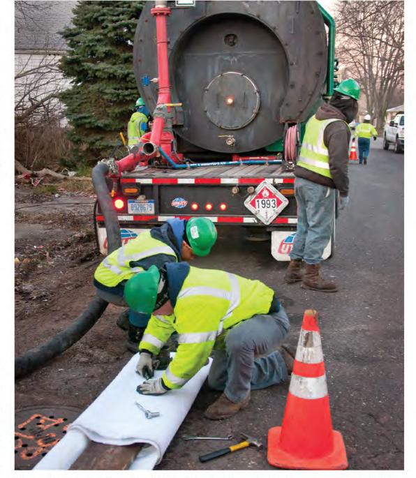
Crew members Kendra Rutgers, left, and Dale Eddy cut a hole in a liner for the air-steam fitting as other crew members set up for the lining job.
