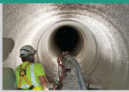
A technician uses IPR's proprietary EcoCast technology on a pipe rehabilitation project. EcoCast is one of several pipe, tunnel and manhole rehabilitation technologies IWPC offers its customers. (Photo courtesy of Inland Waters)
