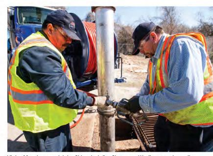
Victor Mendoza and John Shipp install a Stoneage Warthog nozzle on the end of the jetter hose to break up the clog in the drain.
