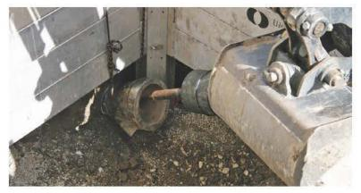
The backhoe bucket pushes down on the 8-inch HDPE pipe to assist the angle of entry. The 8-inch bursting head is designed to slide forward. Once the pull began, the polyethylene cap and pipe caught up with it.
