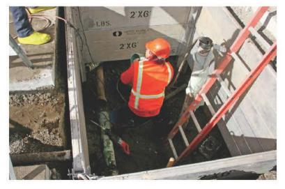
A Therma worker in the shoring box removes a section of 6-inch PVC pipe where it connects to the 4-inch cast iron pipe running 185 feet into the plant. They have already cut the 2-foot-wide slot in the concrete in preparation for the first pull. adjacent underground supply lines. They cut a hole in the manhole wall opposite the inlet pipe, enabling the cable to pass through the pulling pit, and enlarged the inlet more than 12 inches to enable the bursting head to enter.
