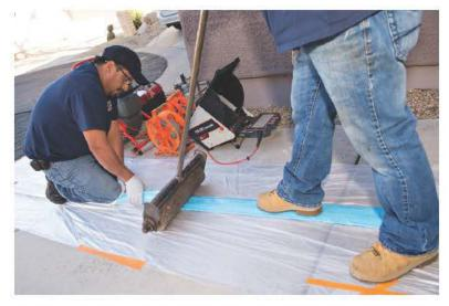
ABOVE: Raul Lopez, left, and Ramon Martinez use a roller to fully impregnate the liner with epoxy prior to installation in the 4-inch pipe. RIGHT: Lopez keeps a firm grasp on the liner while Martinez pours in the epoxy.
