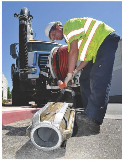
A vacuum truck operator prepares to insert an ENZ USA Ejector nozzle into a 48-inch siphon.
