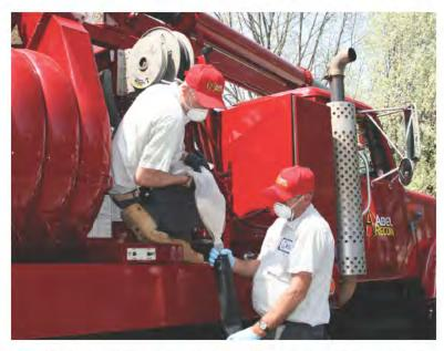
ABEL RECON crew members prepare chemical root control applicator equipment to remove roots from a sewer line.
