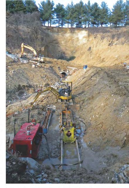
Looking upstream at the jacking pit with the red hydraulic power unit, the auger boring machine and platform sled, mini excavator, and the opening of the 66-inch casing behind it. Underneath it all are 48-inch steel casings to drain water. (Photos courtesy of Glenn Grove)
