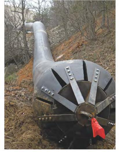
The team excavated a pulling pit 150 feet further downstream, then poured a concrete pad reinforced with steel plates to withstand pressures greater than 400,000 pounds from the 48-900 auger boring machine (American Augers) and platform sled (Michael Byrne Mfg.). They parked a Komatsu mini excavator on the slab to handle 15-foot-long DD50 directional drill steels.
