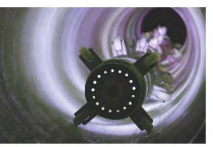
The UV light train rolls through a fiberglass-lined pipe during the curing process.
