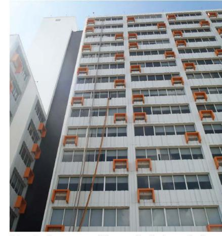
Air hoses from the compressor and dryer run up the side of an apartment building to the eighth-floor control room. Clear hoses coming down from the 15th floor go to the separator and dust collector. (Photos courtesy of Florida Pipe-Lining Solutions)
