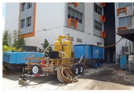
The Atlas Copco 1100 air compressor pushes air through the Ingersoll-Rand desiccant dryer to remove any moisture from the pipes before lining.
