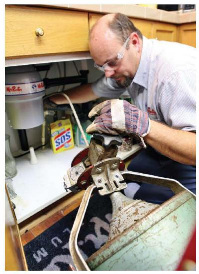
Shaylin King uses a Spartan cable machine to clean out a kitchen sink drain
