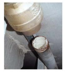
A 2-inch trunk line with a 16-mil ANSI/ NSF Standard 61-certified epoxy coating.
