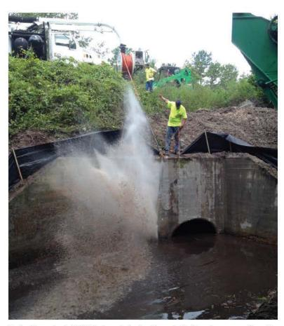
Technician Jody Wright signals technician Josh Knowles, operating the GapVax MC-1510 combination vacuum truck, to pull back on the jet hose. Wright uses a tiger tail to protect the hose from scraping against the concrete as he cleans the barrels with a C-Ray sewer nozzle from NozzTeq. (Photos courtesy of Engineered Lining Systems)
