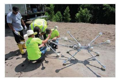
ABOVE: ELS workers assemble the Double Core 10-foot-long UV light train with eight 1,000watt UV bulbs, four forward and four aft between the sets of legs. RIGHT: Workers formed a nose on the SAERTEX fiberglass-reinforced plastic liner and added a pulling collar. The 2-mm-thick gliding foil beneath the liner protects it and facilitates its passage.
