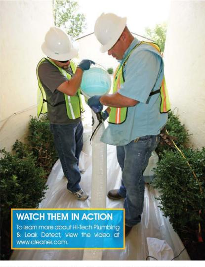
ABOVE: Vice president Matt Amick, left, and Nu Flow specialist Mark Wheaton fill a Nu-Flow system bladder with epoxy before repairing a sewer main in Edmond, Okla. BELOW: Wheaton rolls out a Nu Flow system bladder filled with epoxy before repairing a line at an apartment complex in Edmond, Okla.
