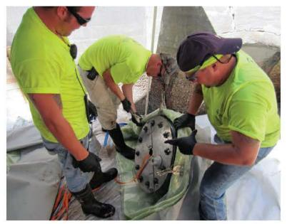
Left to right: Technician Mikal Biegner, project manager Danny Knight, and Jody Wright insert the steel packer at the head of the liner. Pulling the orange line brings the Double Core 10-foot-long UV light train forward.
