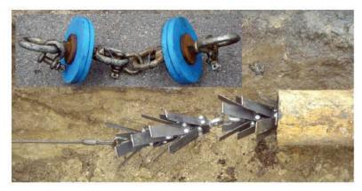
ABOVE: A winch system pulls pairs of clamped custom-made drag scrapers into heating pipes to clean them in Roswell, N.M. Inset: Double sets of squeegee plugs remove tailings. RIGHT: Fusing the 13-foot-long sticks of Climatherm SDR 11 composite pipe from Aquatherm left a weld bead. Workers removed the interior bead using a long pole with a spring-loaded blade that shaved off and extracted the bead. The light blue ring on the end of the pipe is the thermal liner.
