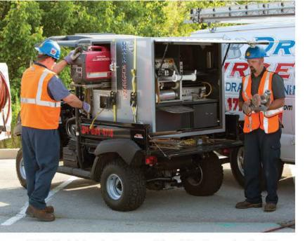
ABOVE: Technicians Joe Donovan, left, and Rico Pozzo set up the ATV generator (Honda) and Envirosight ROVVER 125 inspection camera. RIGHT: Pozzo and Donovan review an inspection video with principal Benji Grimes.
