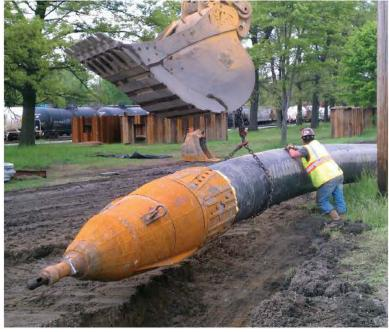
Midwest Trenchless Services employee Jon Snyder assists as the bursting head, skirt expander and 32-inch HDPE pipe are lowered into the pit.
