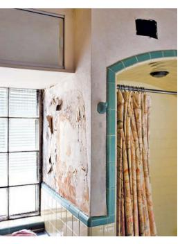
Leaks above the secondfloor master bath and shower caused the concrete ceiling and exterior shower wall to flake and separate. A previous plumber sawed the 4-inch-square hole above the shower stall to expose the west storm drain.
