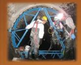
Mainline joints can be tested & sealed with the Logiball Mainline Test & Seal Packers (6"-144" pipe). Packers also available for box culverts & elliptical pipes.
