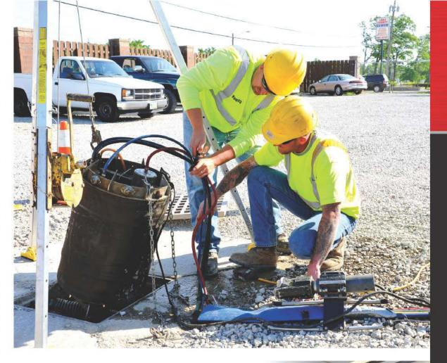
Joe Pennza, left, and Wayne McCloud prepare to lower the grouting unit into a section of sewer. RIGHT: McCloud checks the specific gravity of one of the grouting materials from PYCOSA Chemicals in the truck.
