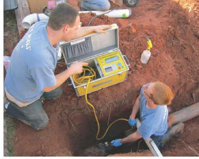
LEFT: Casey Hill uses the Borit tool with 3-inch backreamer bit attached to an industrial drill to widen the channel for feeding the pullback cable to the chain. The communications conduit and two electric lines pass above him. ABOVE: Eric Howell (left) and Casey Hill use the M.T. Deason electrofusion processor to install a HDPE saddle wye.
