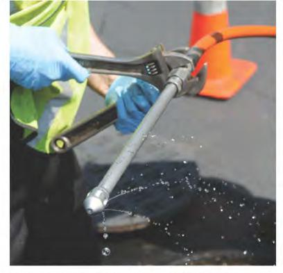
ABOVE: A Standard Enz cleaning nozzle was used to clean storm sewers at Six Flags New England in Agawam, Mass. RIGHT: With the Batman roller coaster in the background, technician Michael Scarfe unwinds the hose from a Harben Hydrojetter on the Six Flags cleaning job.
