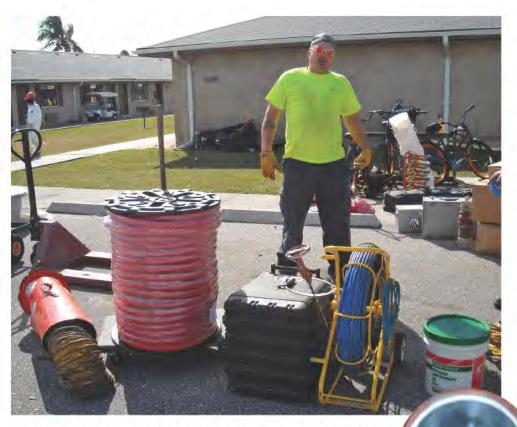
Lining technician Jody Wright rests from unloading material at the job site. Pictured (from left) are the blower used to circulate air, a spool of extra air hose, a pushrod camera system from Ratech Electronics, and Sheetrock mud. Behind him are hand tools and the team's primary mode of transportation, single-speed bicycles. RIGHT: An example of a visually perfect 15-mil epoxy lining in a 1-inch hot water pipe.
