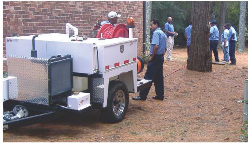
A trailer jetter is used to clean the mainline at an apartment complex.
