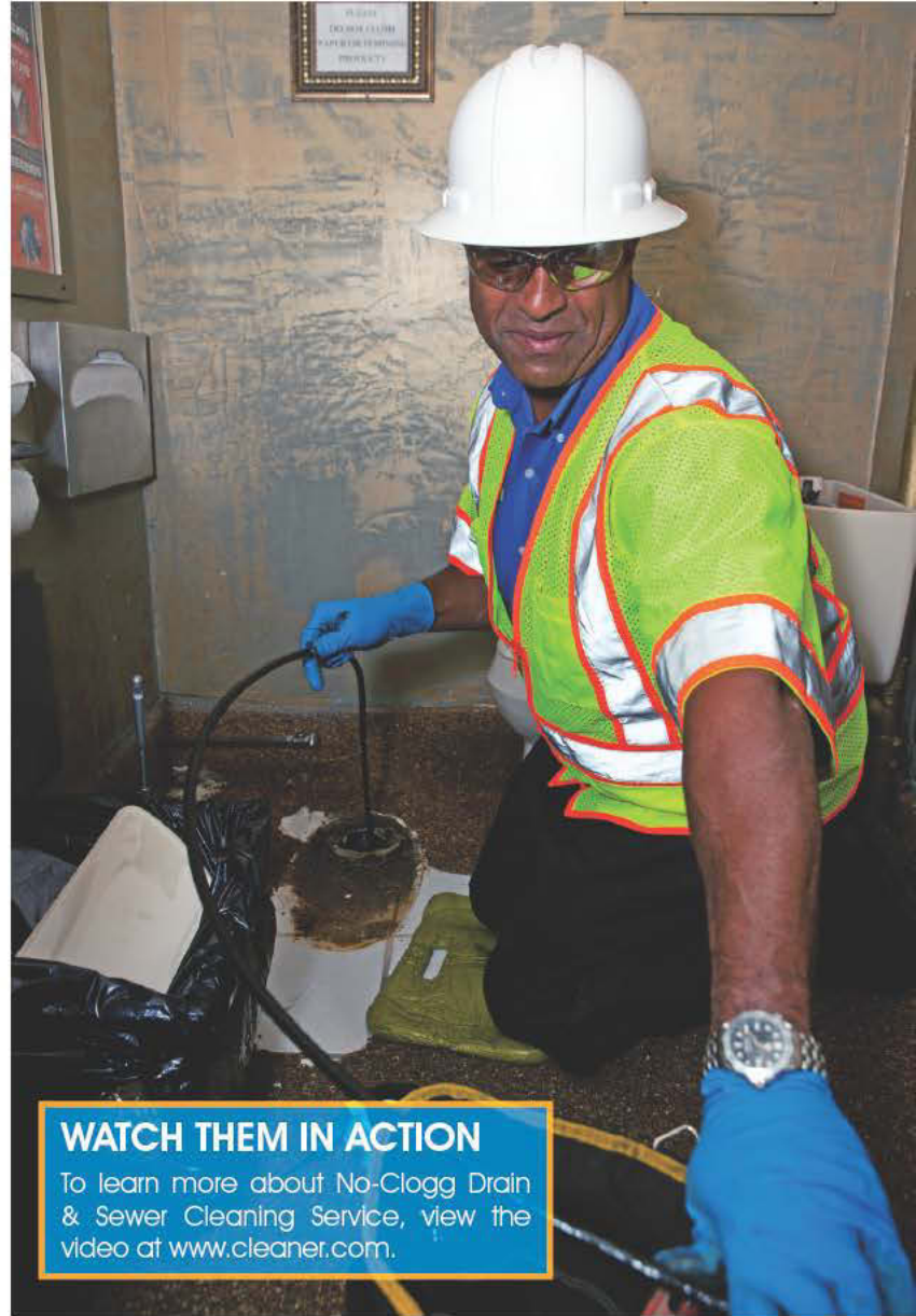
ABOVE: Baron Burems, left, and Juan Ortez feed a new section of pipe into the launching pit on a residential pipe bursting job. RIGHT: After doing a cleaning job a week ago, Burems snakes a drain line to confirm it is still clean. This allows him to give a longer warranty, making his customers happy and ensuring he doesn't have to repeat the work.
