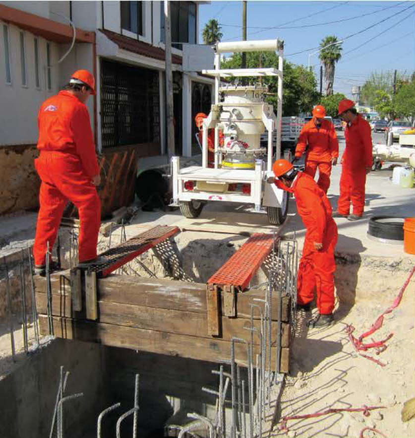
Workers from ACE DuraFlo de Mexico position the Top Gun trailer in line with the steel vehicle ramps over the access pit. A push of a button then activates the wheels to move the trailer forward. (Photos courtesy of Perma-Liner)
