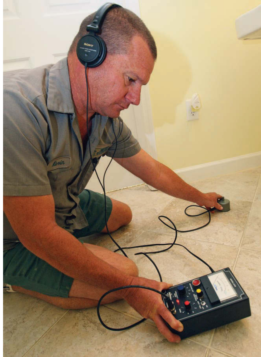
Service technician Kevin Brim uses a MyTana LD30 leak detector on a bathroom inspection. He introduces air into the system, and with the water running, listens for changes in sound under the slab.
