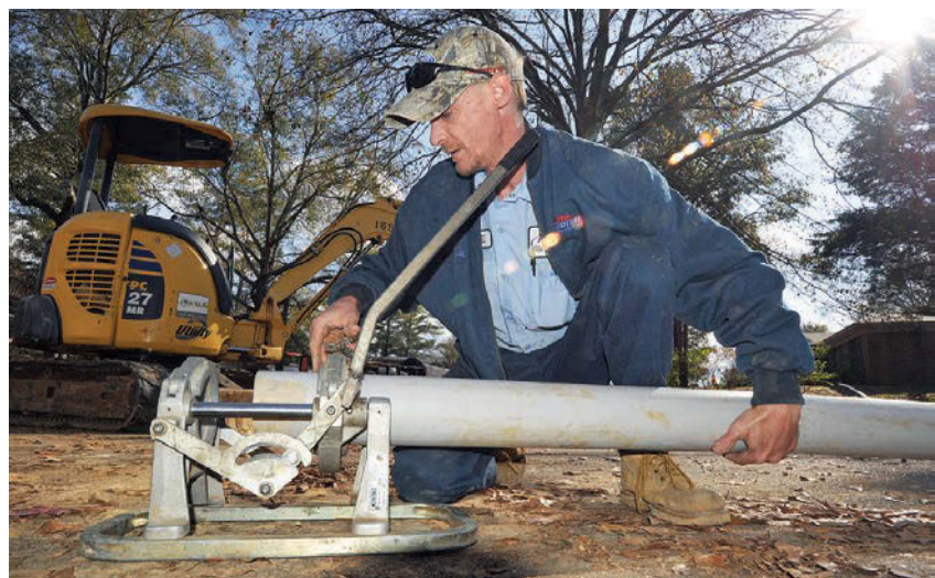
LEFT: Jackson Roto-Rooter employees Michael Hunt (left) and James Gray lower the base for the TRIC Tools pipe bursting equipment into the trench at a home on Beaumont Street in Pearl, Miss. RIGHT: Hunt uses a Central rack system for heat-joining sections of new pipe.
