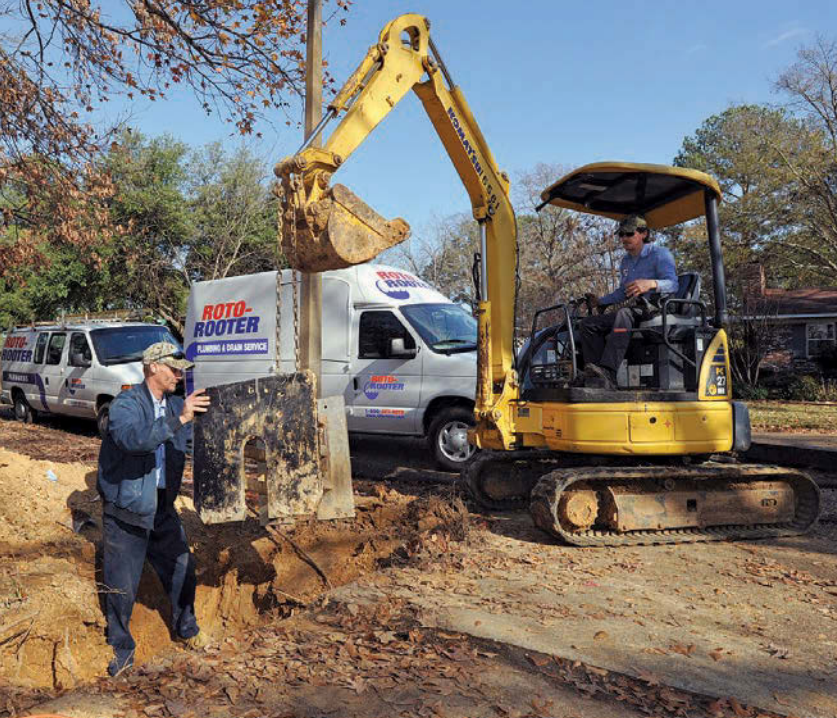
LEFT: Jackson Roto-Rooter employees Michael Hunt (left) and James Gray lower the base for the TRIC Tools pipe bursting equipment into the trench at a home on Beaumont Street in Pearl, Miss. RIGHT: Hunt uses a Central rack system for heat-joining sections of new pipe.
