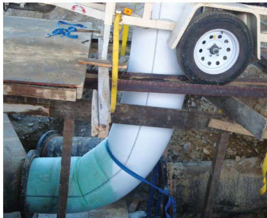
Workers from ACE DuraFlo de Mexico position the Top Gun trailer in line with the steel vehicle ramps over the access pit. A push of a button then activates the wheels to move the trailer forward. (Photos courtesy of Perma-Liner)
