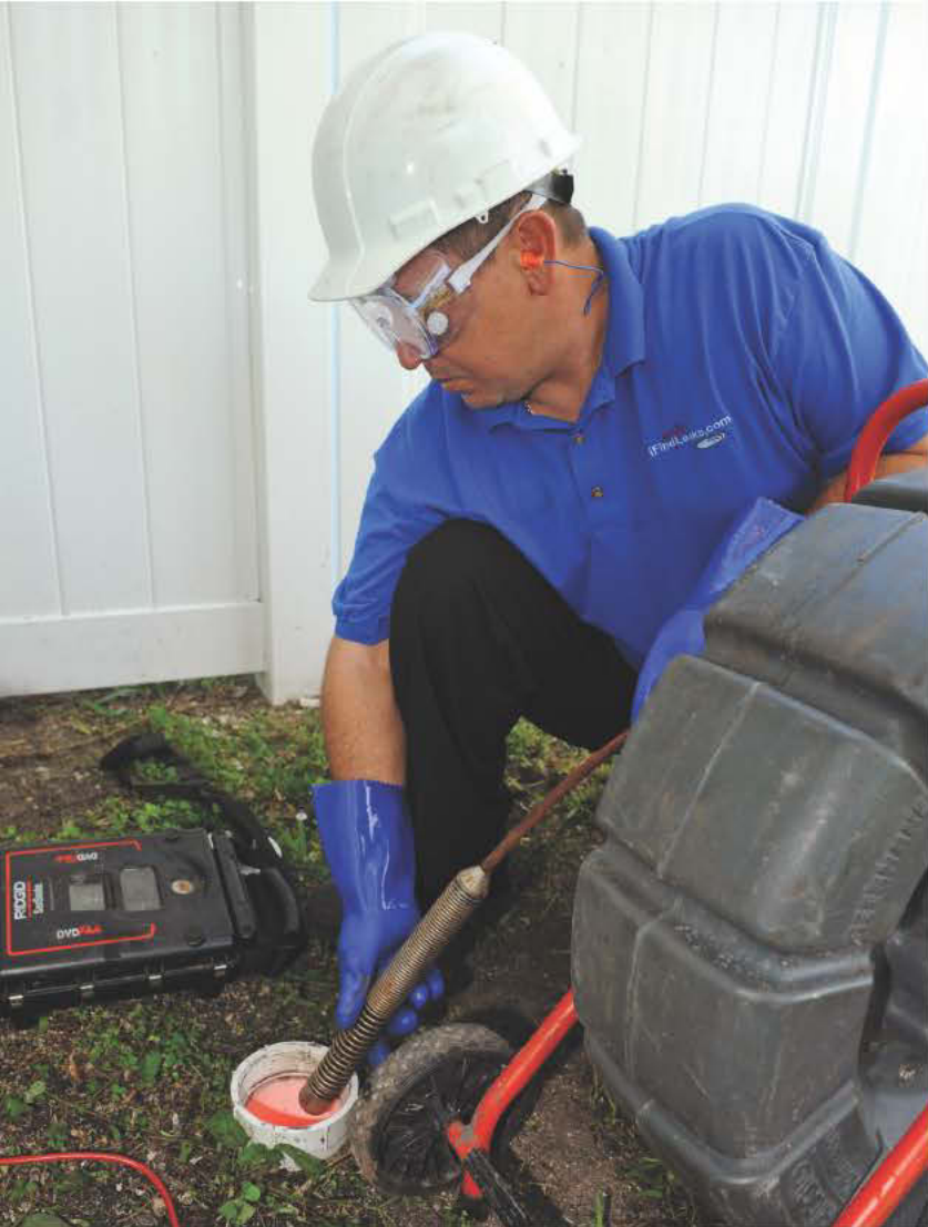
LEFT: Sewer jetting technician Chris Abbott uses a RIDGID SeeSnake to ensure a sewer pipe is clean and clear of debris after jetting. ABOVE: Senior leak locator Dave Richardson uses a FLIR E40bx infrared camera to identify areas of moisture in a bathroom.
