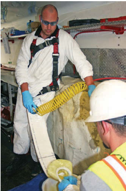
ABOVE: Armand Moinzad guides the winch cable over a pulley as he lowers the lateral launch assembly down the manhole. LEFT: Tony Bergipen (left) and foreman Wayne Powers vacuum impregnate resin into a BLD service connection seal.
