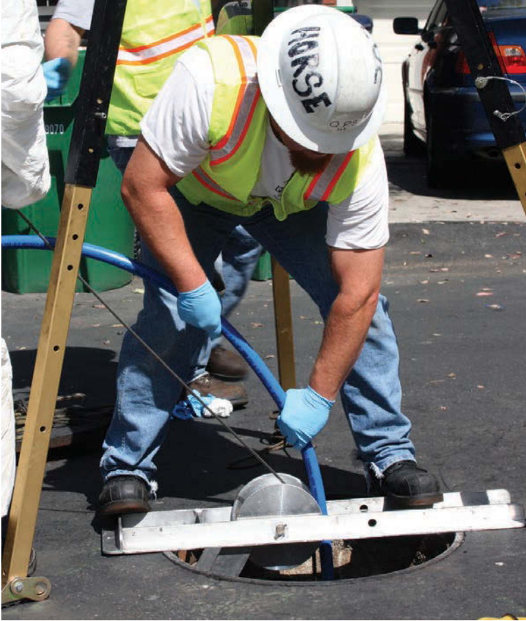
ABOVE: Armand Moinzad guides the winch cable over a pulley as he lowers the lateral launch assembly down the manhole. LEFT: Tony Bergipen (left) and foreman Wayne Powers vacuum impregnate resin into a BLD service connection seal.
