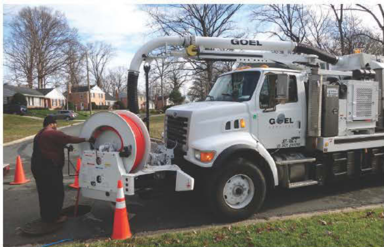
Patrick Johnson of Goel Services Inc. in Washington, D.C., uses the jetter on his Vac-Con combo truck to clean a sewer line in a residential neighborhood in the D.C. metro area.
