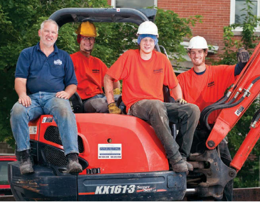
The Utah Pipe Bursting crew includes, from left, Jay Garrett, owner; Brandon Garrett, foreman; Trevor Garrett, laborer; and Matthew Gross, laborer.
