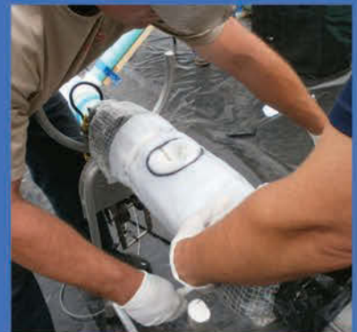
InnerSeal™ Innerwrap™ Lateral Connection Seal
