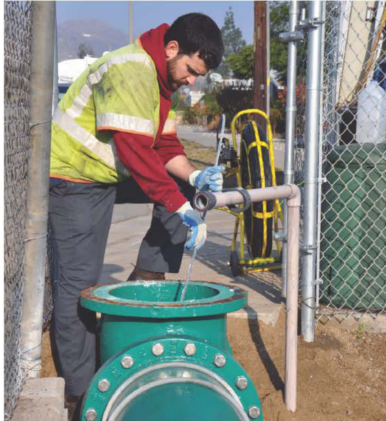
Robert Hueners runs a camera into a 16-inch brine line. Approaching jobs with a sense of urgency helps maximize production.
