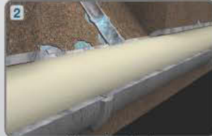
Liner installed
