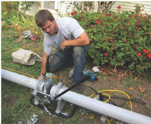
John Sumner fuses another stick of 4-inch SDR-17 HDPE pipe.
