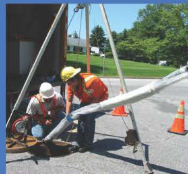
Sectional Main Line Point Repair™
