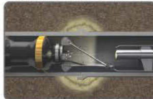
Grout collar stops infiltration
