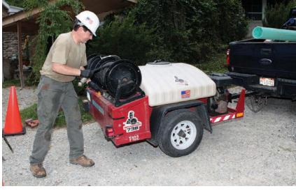
LEFT: Charles Menkhaus helps feed the Perma-Liner into the Perma-Verter. RIGHT: Menkhaus pulls the line from the Spartan trailer jetter to power wash the sewer line prior to lining.
