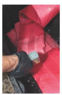
Charles Menkhaus checks the temperature of the Perma-Liner in an ice bath where it is kept cool to prevent hardening.
