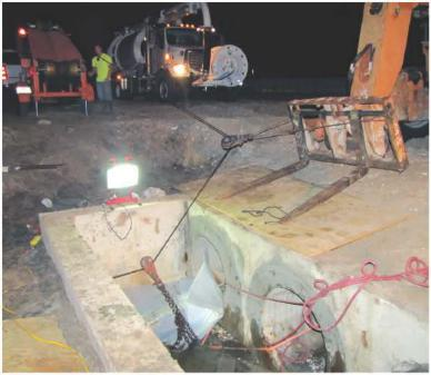
An elaborate winch system involving blocks, the forklift, and an adapted bucket machine pulled the liner into the pipe.
