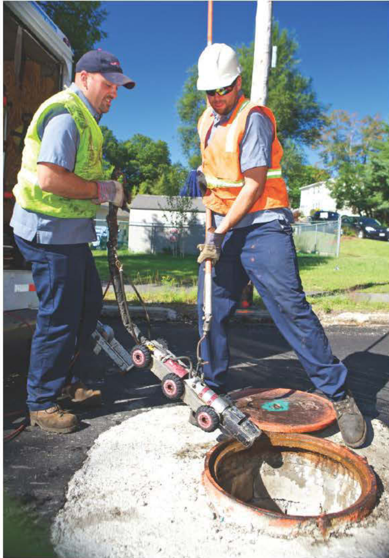
LEFT: Jason Langlais, left, and Christopher Daigle pull the Aries camera out of a manhole after inspection. RIGHT: Jason Langlais operates the Aries camera inspection equipment from inside the CCTV truck.
