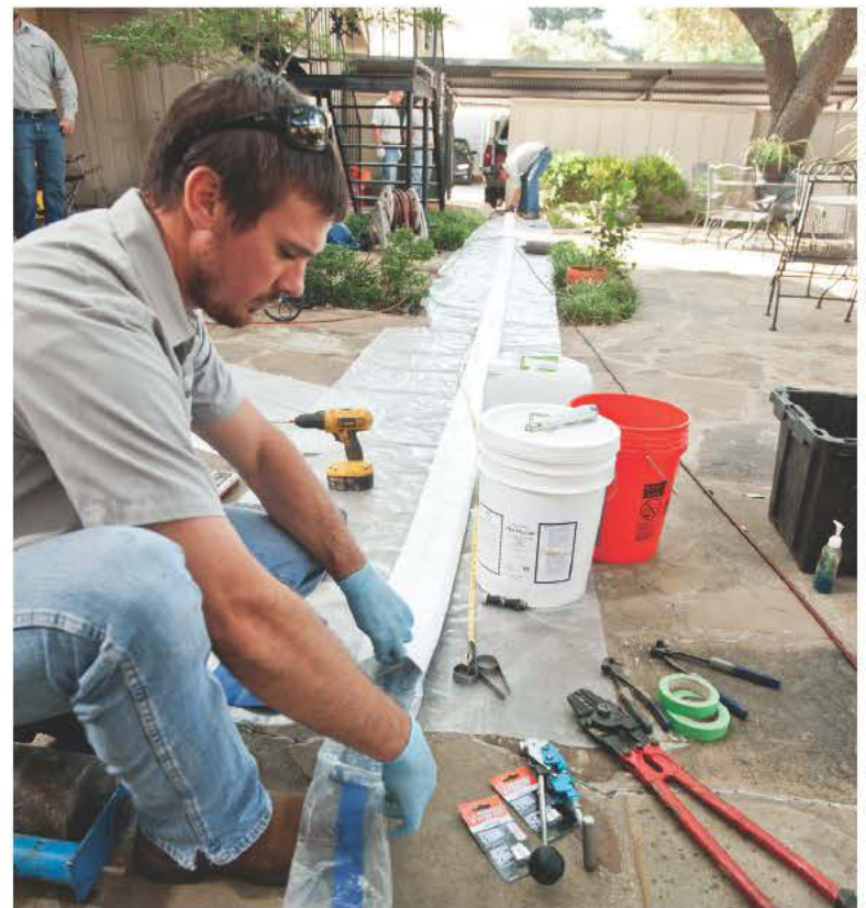
Josh Veach prepares the Nu Flow Trenchless Lining materials.
