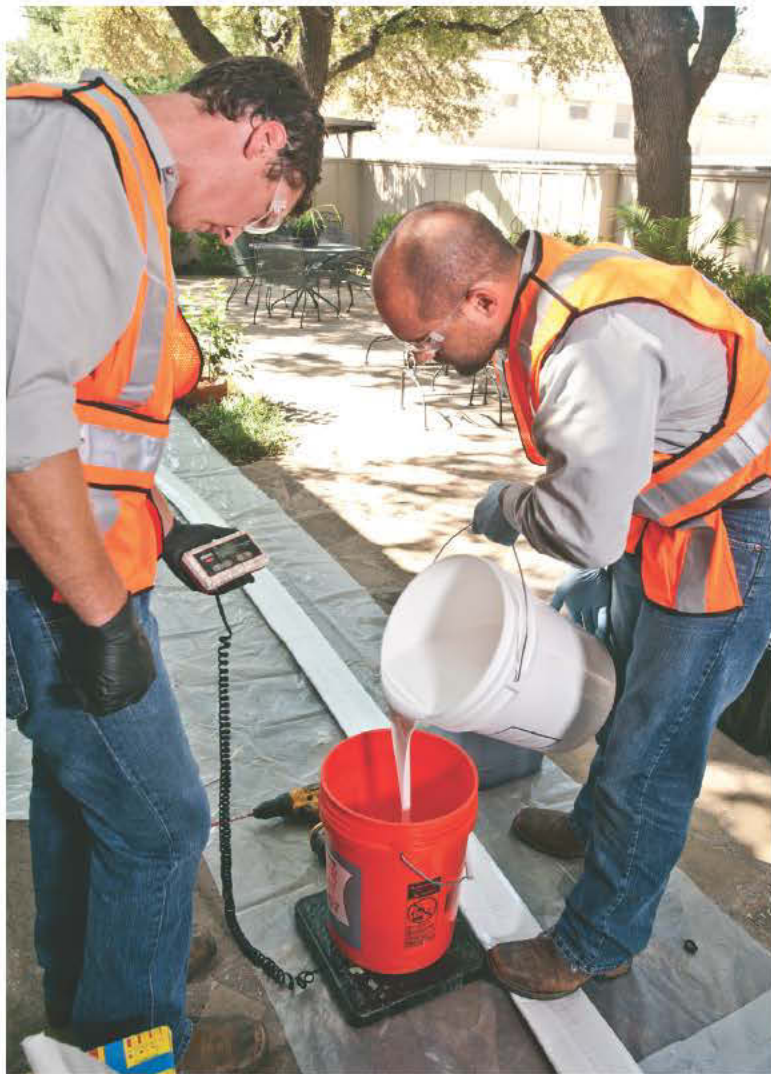
LEFT: Chad Montgomery, left, and Clayton Vitellaro mix cast-in-place epoxy. RIGHT: Josh Veach, Chad Montgomery, Clayton Vitellaro and Casey Van Cleave roll the epoxy mixture through a Nu Flow sleeve.
