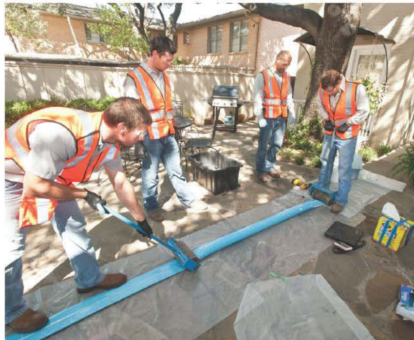
LEFT: Chad Montgomery, left, and Clayton Vitellaro mix cast-in-place epoxy. RIGHT: Josh Veach, Chad Montgomery, Clayton Vitellaro and Casey Van Cleave roll the epoxy mixture through a Nu Flow sleeve.
