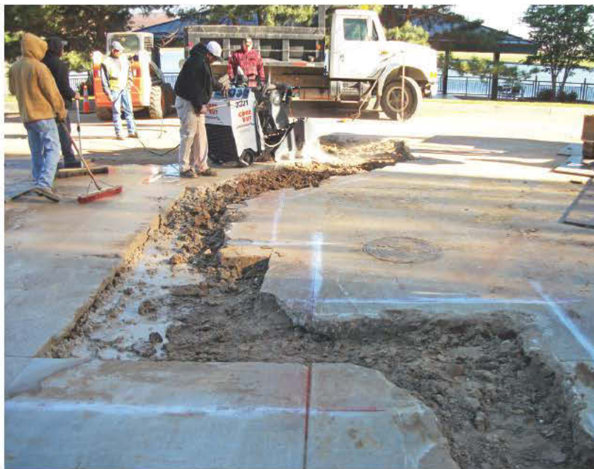
ABOVE: The 350-foot-long replacement pipe snakes over the top of the grease interceptor and under the pickup truck to the entry pit. BELOW: Workers use a self-propelled Core Cut concrete saw from Diamond Products to square excavations in preparation for pouring concrete.
