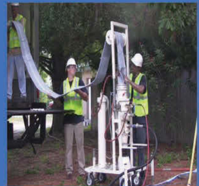
Perma-Main™ Continuous Air Inversion
