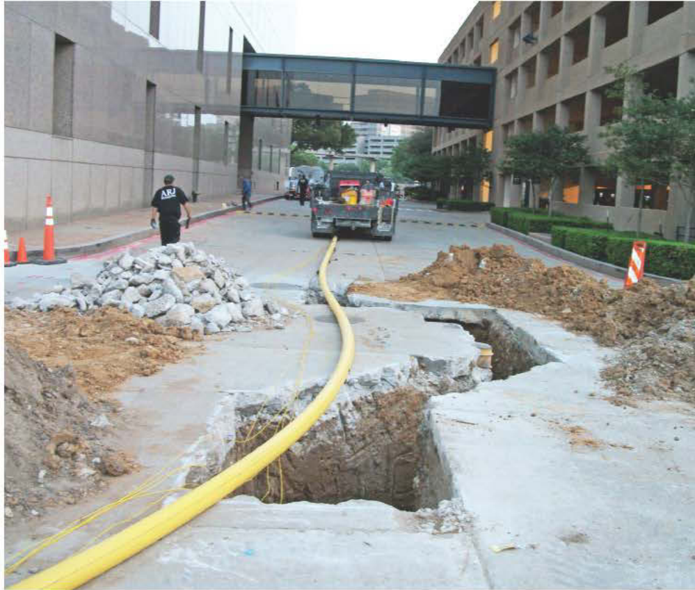
ABOVE: The 350-foot-long replacement pipe snakes over the top of the grease interceptor and under the pickup truck to the entry pit. BELOW: Workers use a self-propelled Core Cut concrete saw from Diamond Products to square excavations in preparation for pouring concrete.
