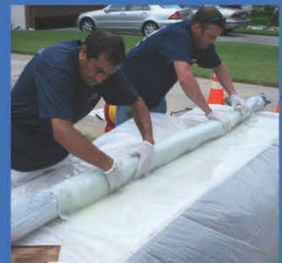
Sectional Main Line Point Repair™
