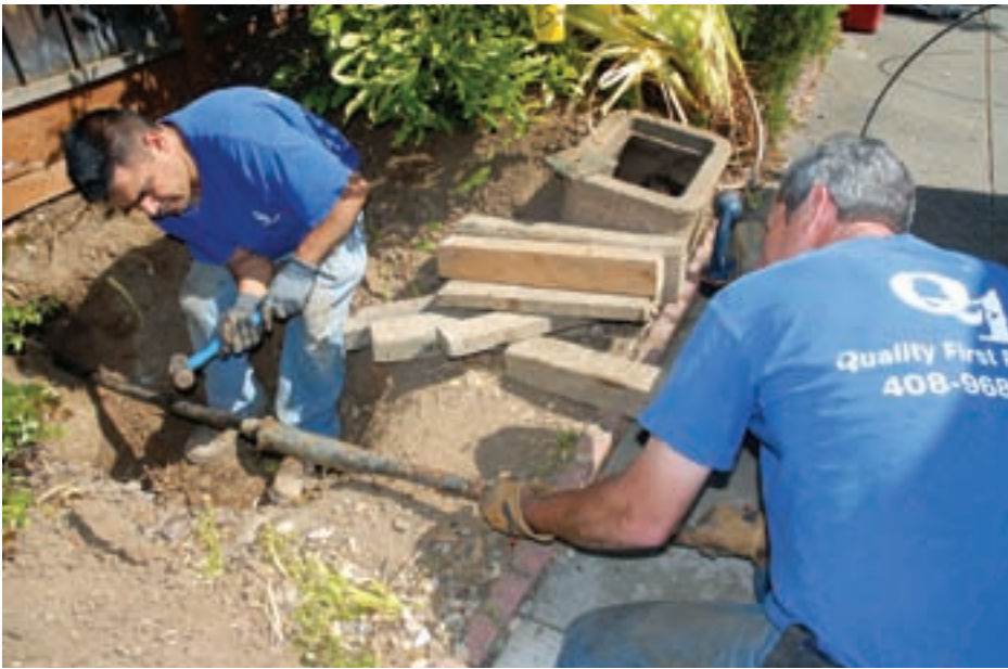
LEFT: Atanacio Francisco hammers the last length of galvanized pipe off the bursting head as Bob Zamaroni hangs on and pulls. The stop plate is on top of the utility box. ABOVE: Pull completed. A 2-inch-long Acme screw adaptor attaches the 1-inch HPDE pipe behind the 16-inch-long bursting head with 6-inch-long slitting blade welded at rear. Note the 2-degree bend in the cable at the swage and the length of the swage before it reaches the inverted slitting blade.
