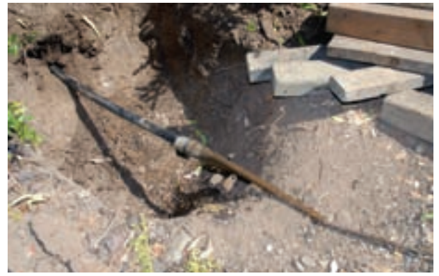
LEFT: Atanacio Francisco hammers the last length of galvanized pipe off the bursting head as Bob Zamaroni hangs on and pulls. The stop plate is on top of the utility box. ABOVE: Pull completed. A 2-inch-long Acme screw adaptor attaches the 1-inch HPDE pipe behind the 16-inch-long bursting head with 6-inch-long slitting blade welded at rear. Note the 2-degree bend in the cable at the swage and the length of the swage before it reaches the inverted slitting blade.
