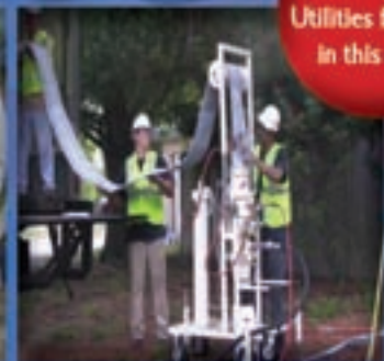
Perma-Main™ Continuous Air Inversion
