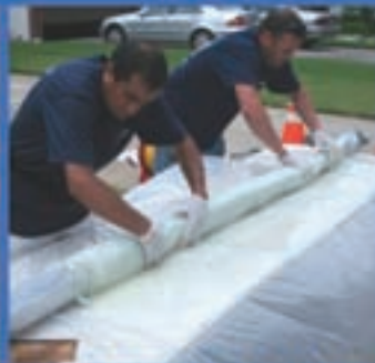
Sectional Main Line Point Repair™
