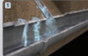
Leaking lateral
