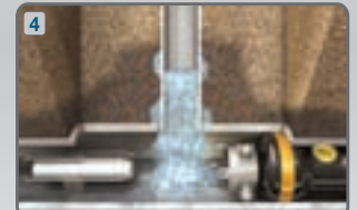
Water infiltration at lateral
