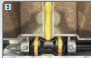
Lateral packer injecting grout
