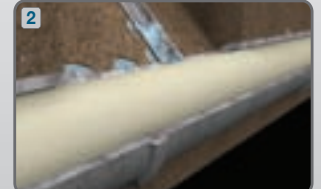
Liner installed
