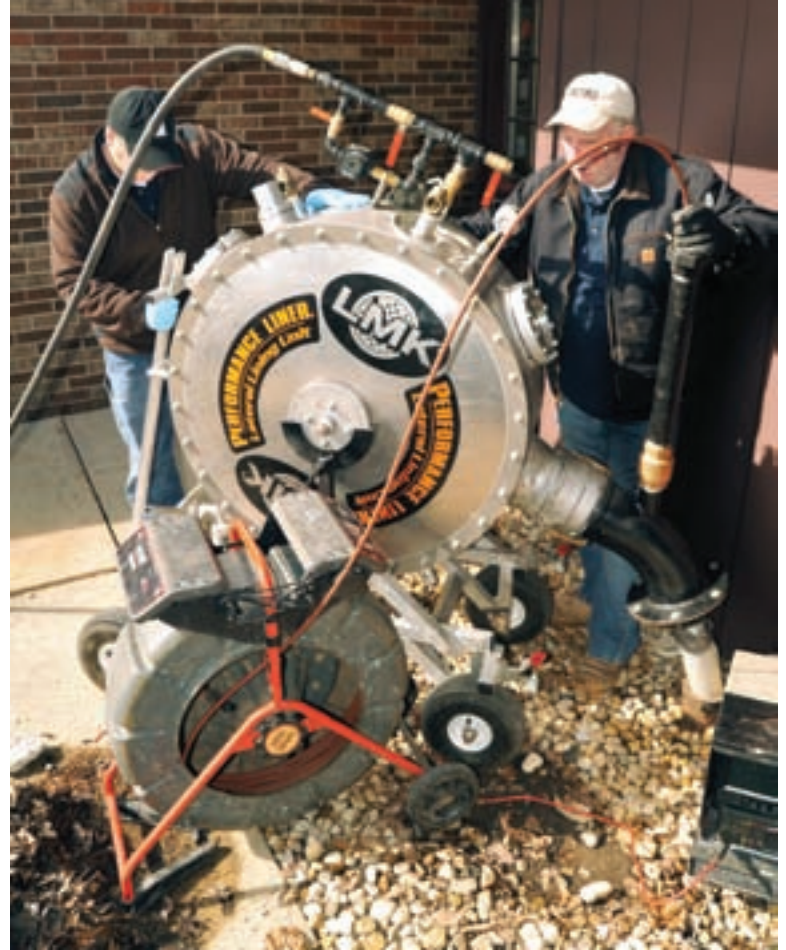
TOP: Chris Jacobs, left, and owner Jake Saltzman unload the Big Brute cart jetter. RIGHT: Owner Jake Saltzman, left, and his father, Jeff Saltzman, use a RIDGID SeeSnake camera and the LMK Technologies system on a lateral lining job.
