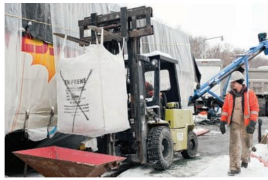
Mike Shantz helps transport the filter aid (ENPRENE from En Chuan Chemical Industries) for dewatering. The solids will go to a landfill or to a compost facility.
